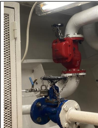
Photo #11 8/7/23 Image: IMG_0620 By: Dobrowski Description: overboard discharge lock
