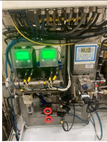
Photo #05 10/1/23 Image: IMG_E0786 By: Dobrowski Description: OWS oil content meter
