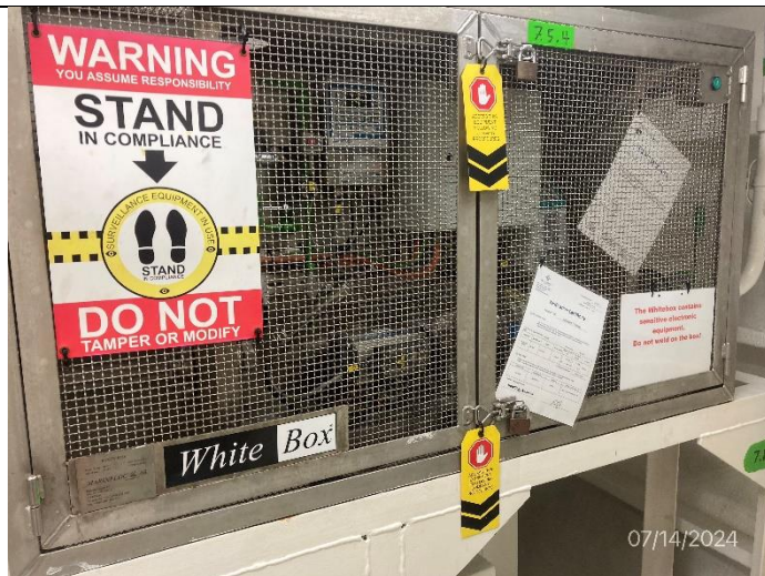
Photo # 19 Image: IMG_1841 Date: 7/14/2024 Taken by: Evan Dobrowski Description: Photo showing double locked marinfloc white box system.
