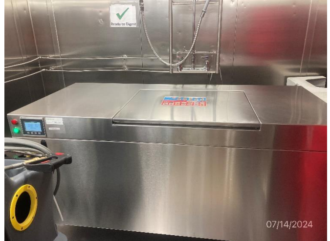
Photo # 2 Image: IMG_1798 Date: 7/14/2024 Taken by: Evan Dobrowski Description: Photo of Bi Hi-Tech Digester
