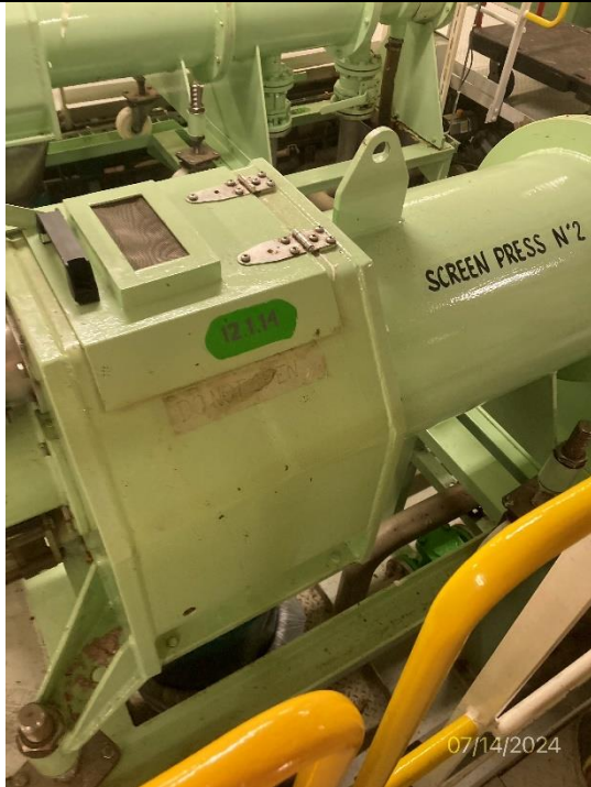
Photo # 15 Image: IMG_1824 Date: 7/14/2024 Taken by: Evan Dobrowski Description: Photo of Wartsila MBR system Screen Press.
