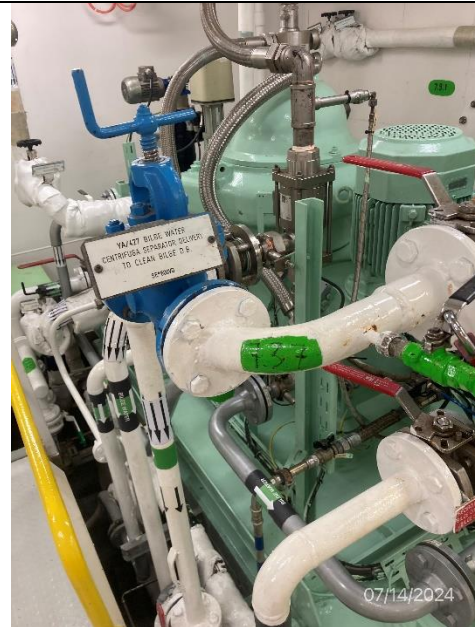
Photo # 18 Image: IMG_1838 Date: 7/14/2024 Taken by: Evan Dobrowski Description: Photo showing bilge water centrifugal separator.
