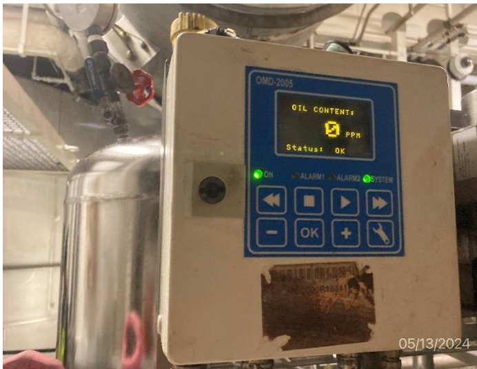
Photo # 15 Image: IMG_1531 Date: 5/13/2024 Taken by: Evan Dobrowski Description: OWS continuous monitor
