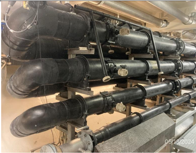
Photo # 5 Image: IMG_1521 Date: 5/13/2024 Taken by: Evan Dobrowski Description: Hydrotech filtration component
