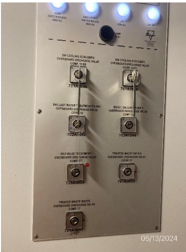
Photo # 11 Image: IMG_1527 Date: 5/13/2024 Taken by: Evan Dobrowski Description: Discharge valve lockout system
