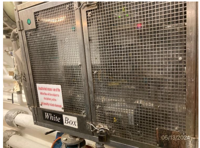
Photo # 16 Image: IMG_1532 Date: 5/13/2024 Taken by: Evan Dobrowski Description: Whitebox
