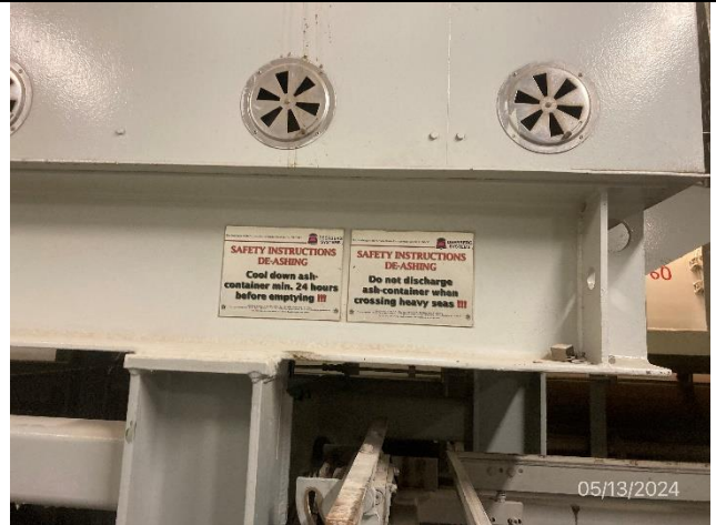
Photo # 18 Image: IMG_1534 Date: 5/13/2024 Taken by: Evan Dobrowski Description: incinerator ash collection point
