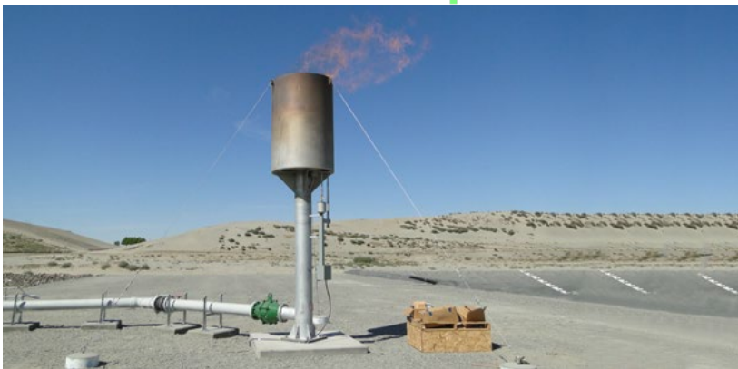
Figure 1. Example of the Open Flare type used at the Ephrata MSW Landfill.
