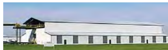
Single-pass reversing dryers are built with individual fans and burners for custom drying per bin.
