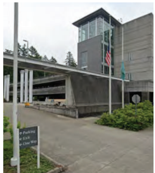
Entrance to parking at ECY Headquarters Building
