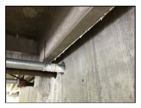
**Photo 1**: Water seeping through the concrete upper parking deck washing the minerals out of the structural concrete elements weakening the overall structure.
