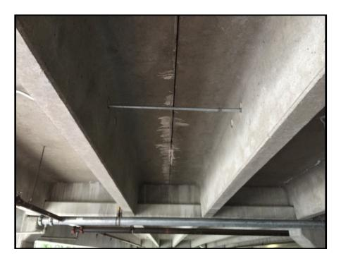
**Photo 4:** Joints between precast structural members showing water intrusion. Continued intrusion. Will cause failure of the joint.
