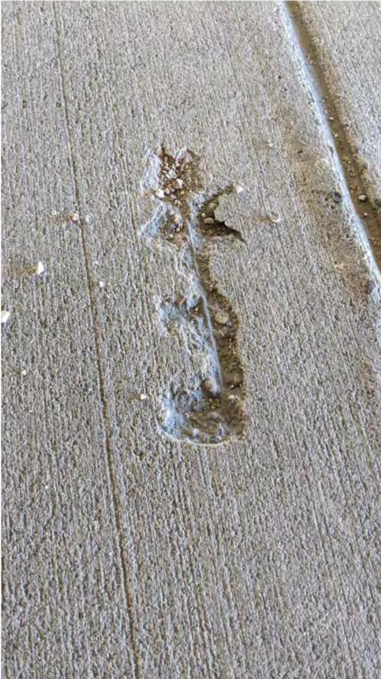
Figure 18 - Minor Deck Spall with Exposed Reinforcing
