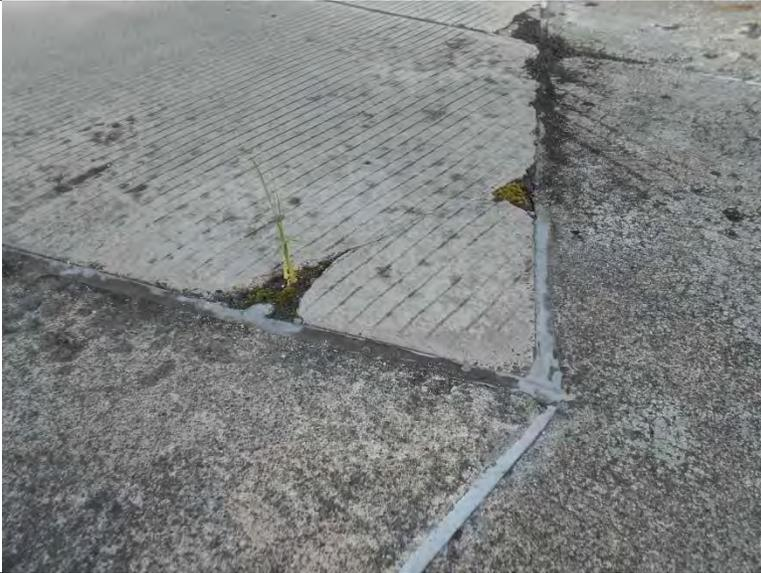
Photograph 19: Overview image showing topping layer deterioration, organic growth in divots.
