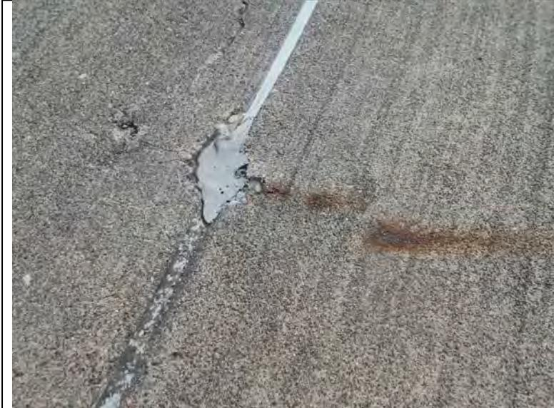
Photograph 23: Detail from previous image showing deterioration of joint edge and exposed and corroding reinforcing steel.
