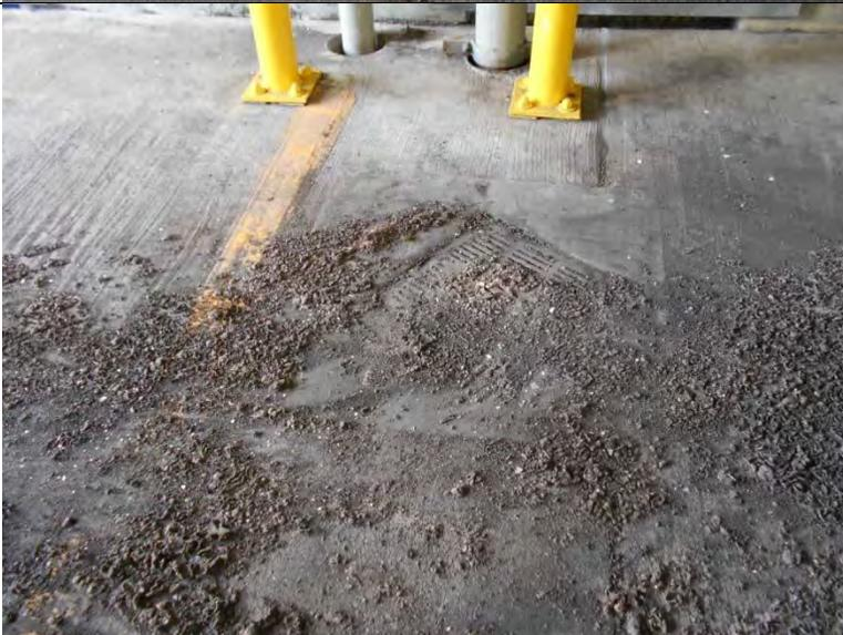
Photograph 27: Detail from previous image showing accumulation of sediment and debris at drain grate. Regular maintenance should include clearing of debris from drainage pathways.
