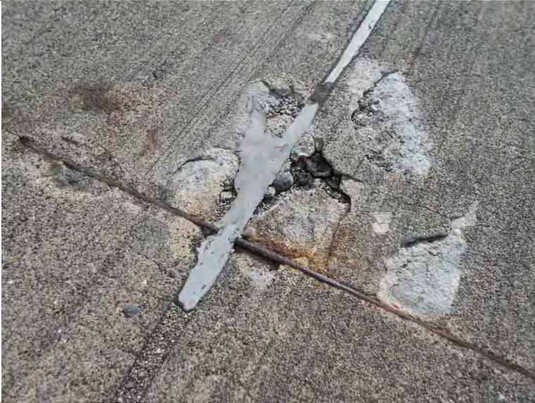
Photograph 25: Detail from previous image showing deterioration of joint edge and exposed and corroding reinforcing steel.
