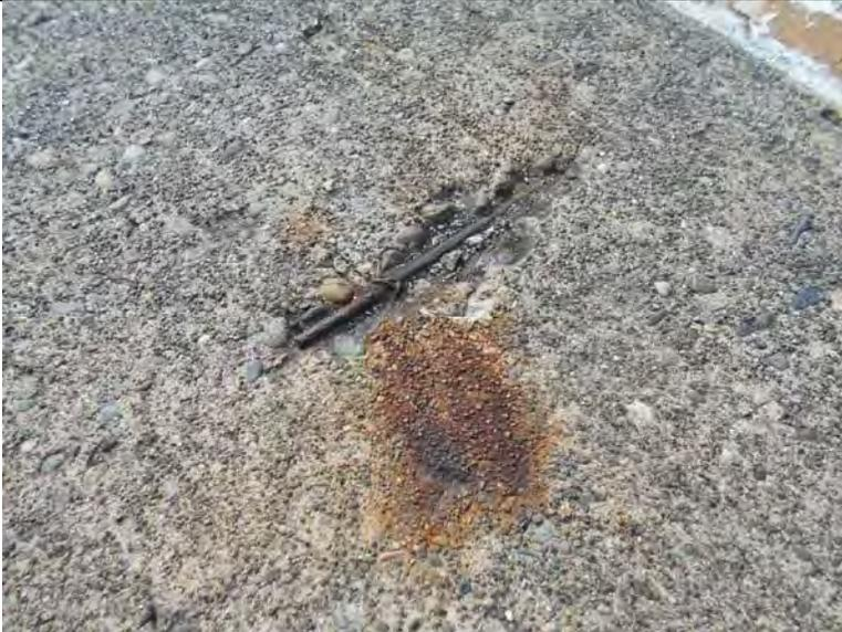
Photograph 20: Exposed and corroding reinforcing steel.
