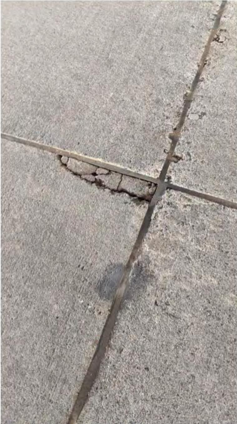
Figure 13 - Deck Crack at Intermediate Joint
