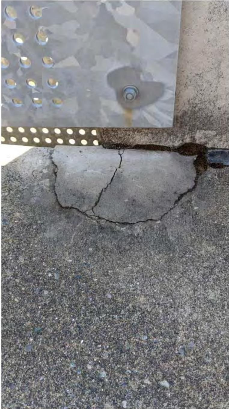
Figure 15 - Deck Cracking at Walls
