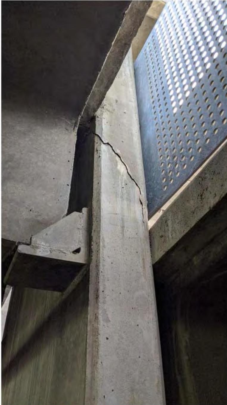
Figure 11 - Center Wall Diagonal Crack
