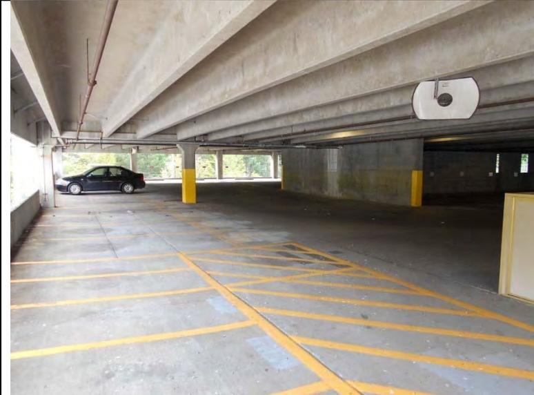
Photograph 5: Overview of the precast double T configuration.
