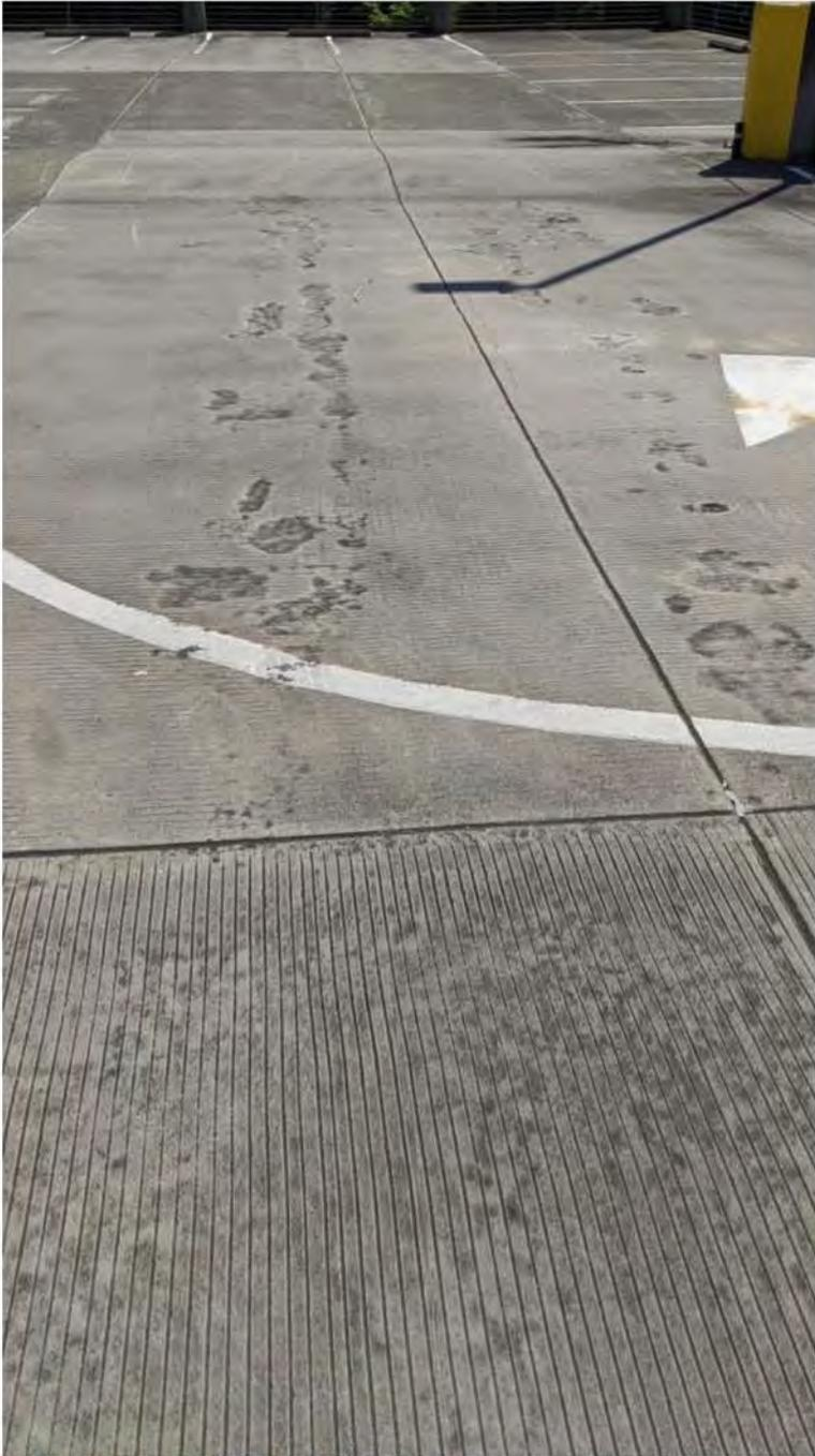
Figure 23 - Water Stained Low Spots in Overlay
