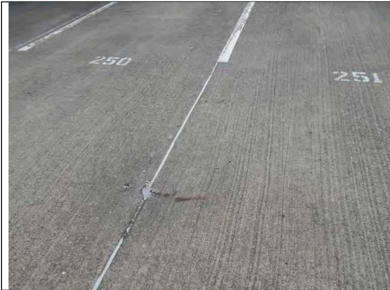
Photograph 22: Typical sealant joint overview.
