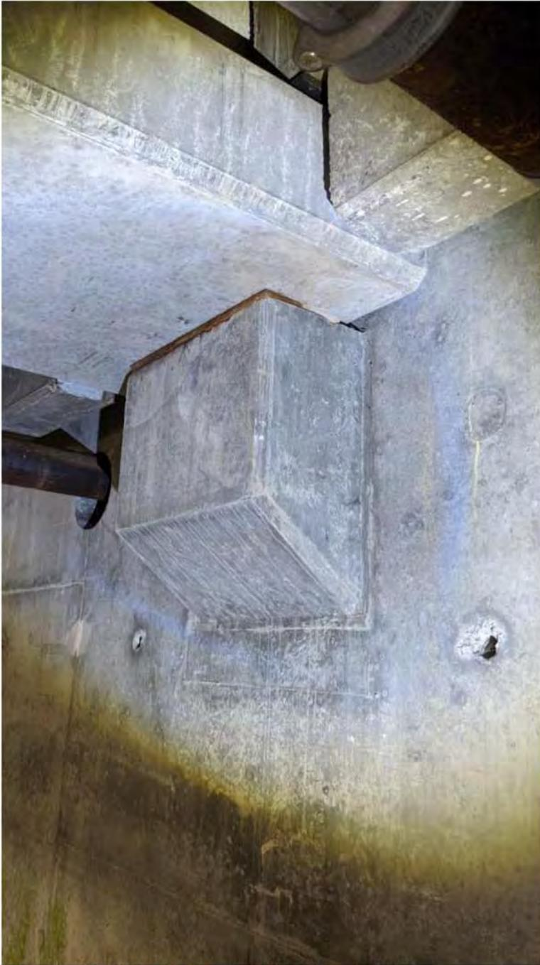
Figure 5 - First Floor Corbel - South End of Garage
