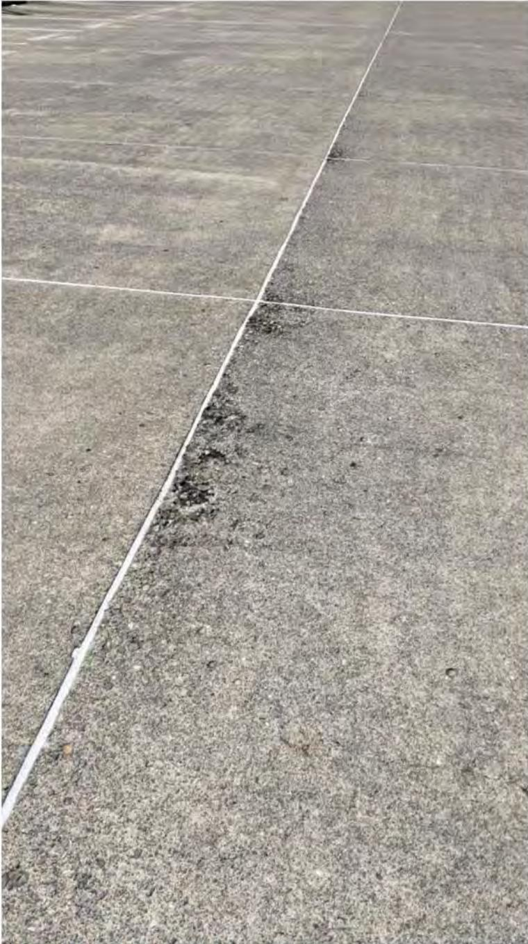
Figure 20 - Deck Spalling and Aggregate Exposure
