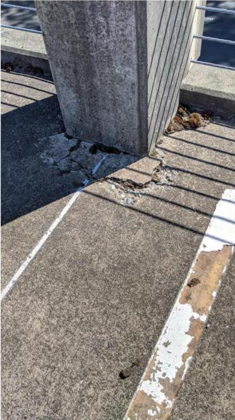
Figure 14 - Deck Cracking at Columns
