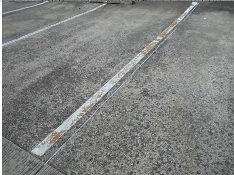
Photograph 15: Typical sealant joint overview.
