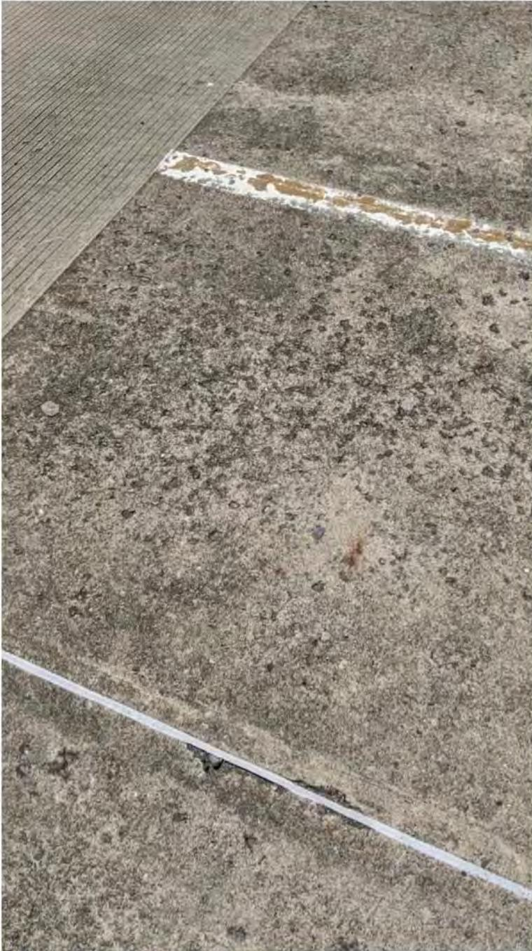
Figure 21 - Deck Aggregate Exposure
