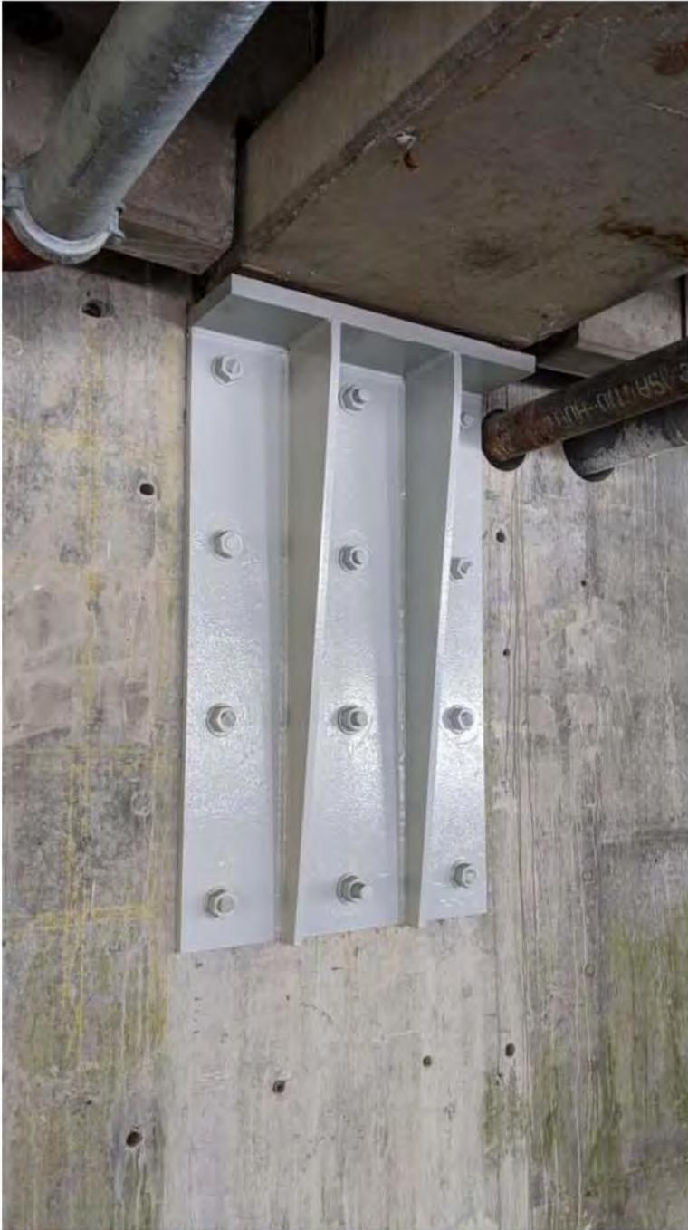
Figure 25 - New North Corbel Supporting Upper Level Girder
