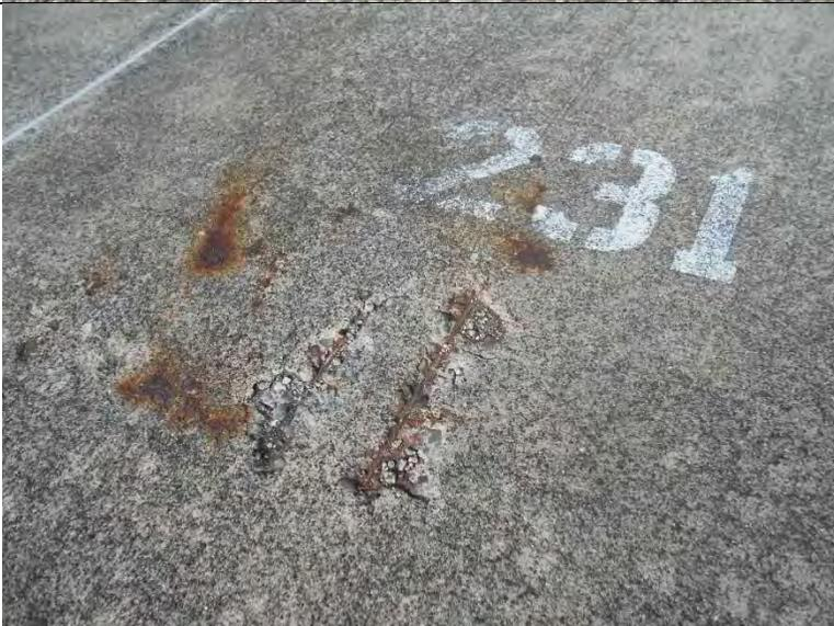
Photograph 21: Exposed and corroding reinforcing steel.
