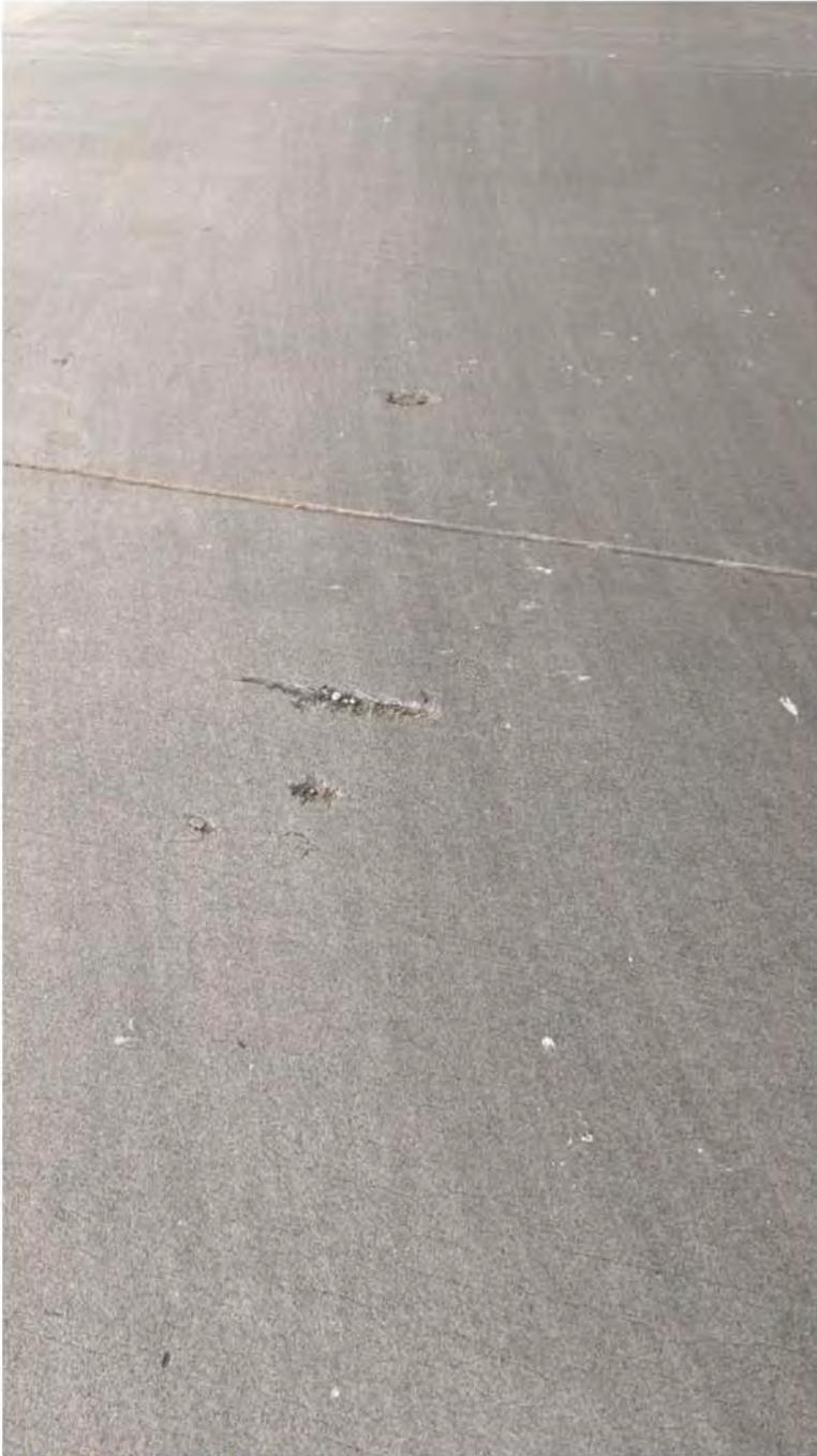
Figure 17 - Minor Spalls in Deck
