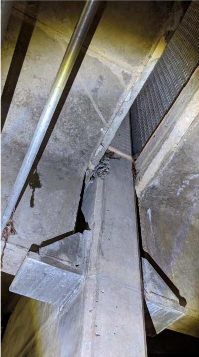
Figure 10 - Center Wall Minor Spalling
