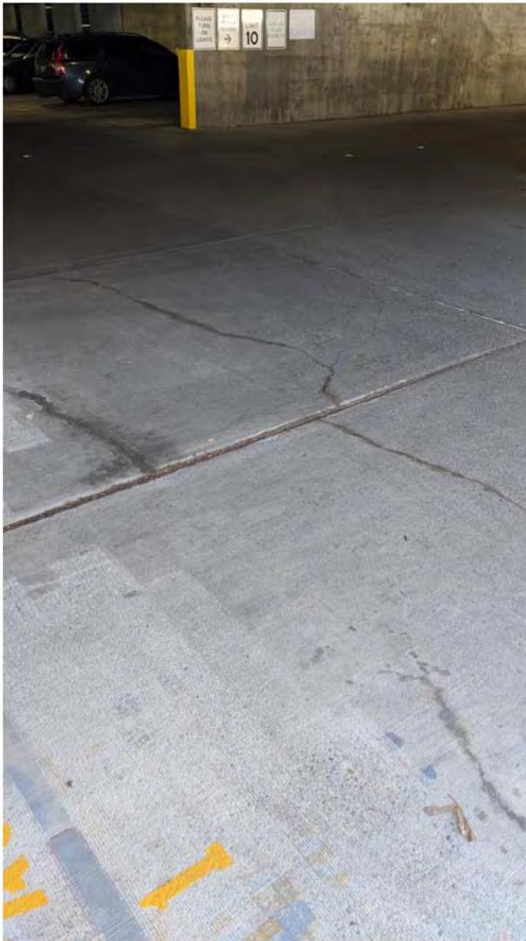
Figure 12 - Deck Cracking at North Entry
