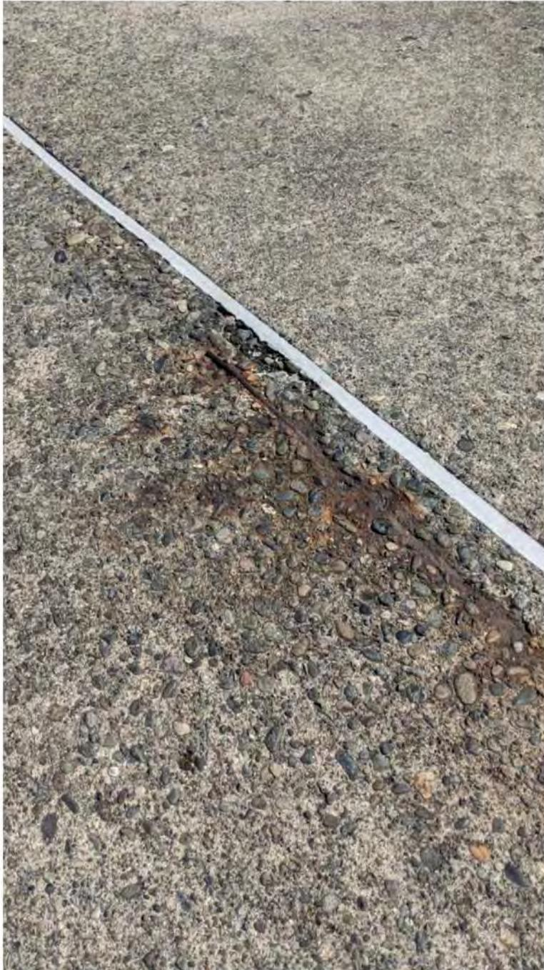
Figure 19 - Exposed, Rusty Reinforcing and Deck Aggregate Exposure
