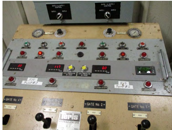
Figure 8 – Hydraulic Control Panel
