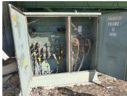
Figure 33 – Existing Pad-Mount Transformer with Doors Open
