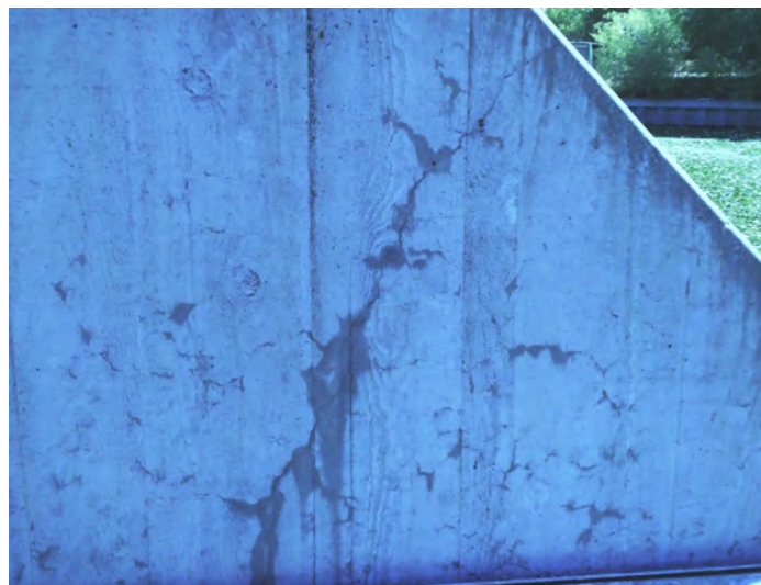
Figure 3 – Showing Crack in East Wall Downstream End
