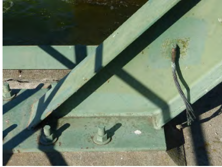
Figure 31 – Grounding Cable Exothermic Welded to Structure
