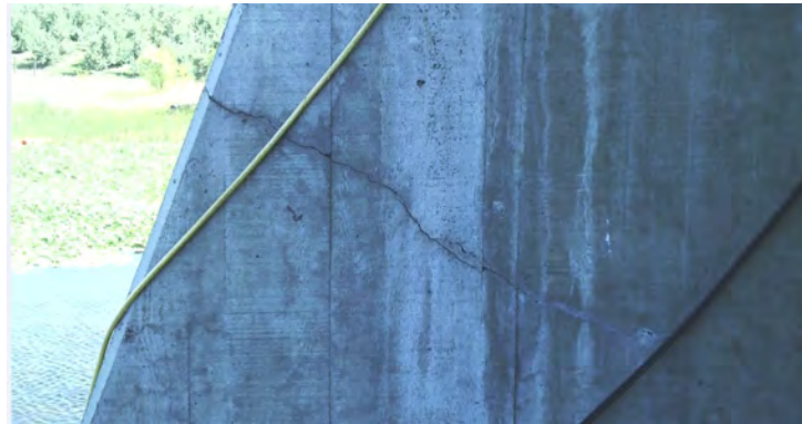
Figure 2 – Showing Crack in East Wall Upstream End
