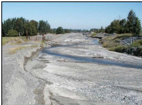
Landslide material in Swift Creek containing naturally-occurring asbestos
