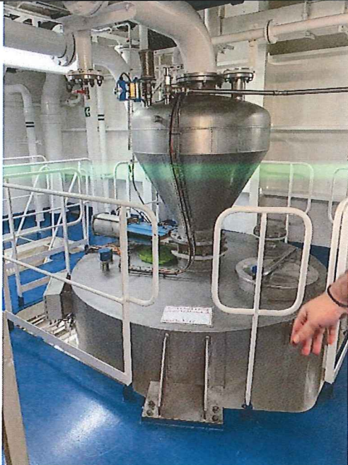
Photo # 25 Image: IMG_0133 Date: 9/9/2021 Taken by: Amy Jankowiak Description: Food Waste Collection tank
