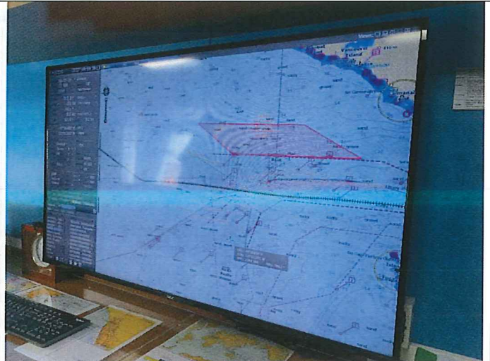
Photo # 2 Image: IMG_0099 Date: 9/9/2021 Taken by: Amy Jankowiak Description: Bridge – Navigation map
