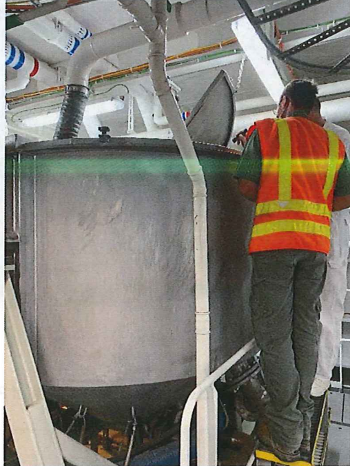
Photo # 6 Image: IMG_0110 Date: 9/9/2021 Taken by: Amy Jankowiak Description: Scanship – Dissolved Air Flotation (DAF)
