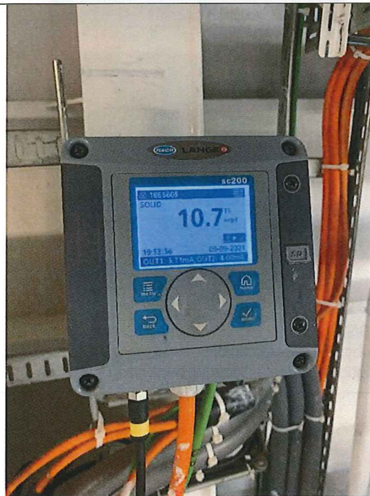
Photo # 8 Image: IMG_0114 Date: 9/9/2021 Taken by: Amy Jankowiak Description: Scanship – TSS reading
