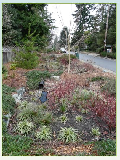
Piped inlet from upslope BMP
