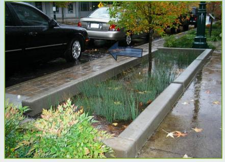
Exit Curb Cut Trench Drain
