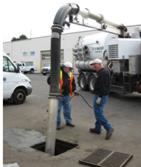
Vactor truck crew cleaning out a catch basin.
