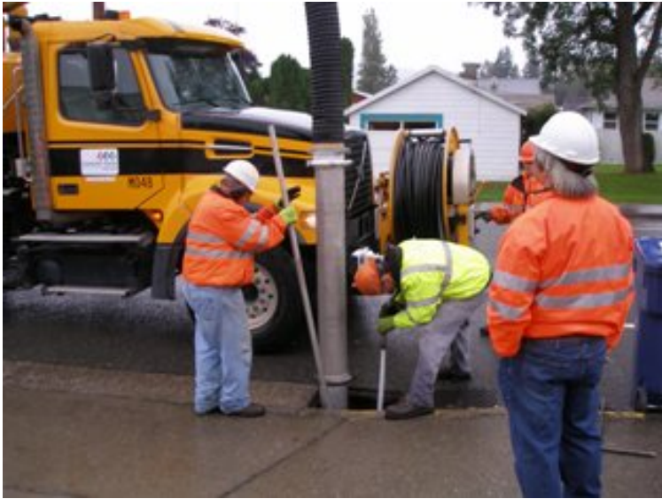
Vactor truck crew dislodging accumulated catch basin solids during cleaning.
