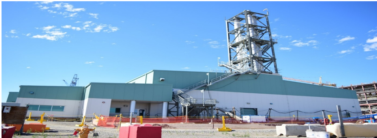
Analytical Laboratory at the WTP facility
