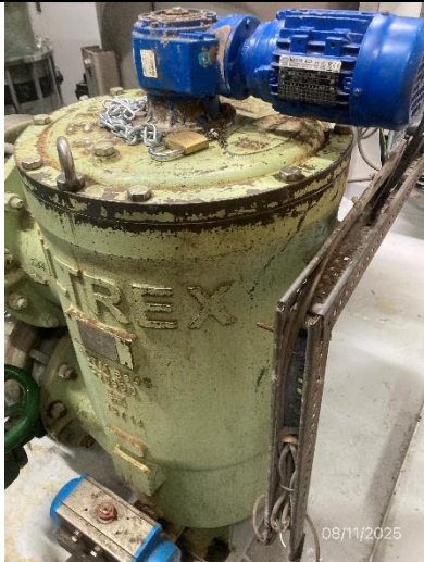
Photo # 17 Image: IMG_2969 Date: 8/11/2025 Taken by: Evan Dobrowski Description: Photo showing food waste biodigester.
