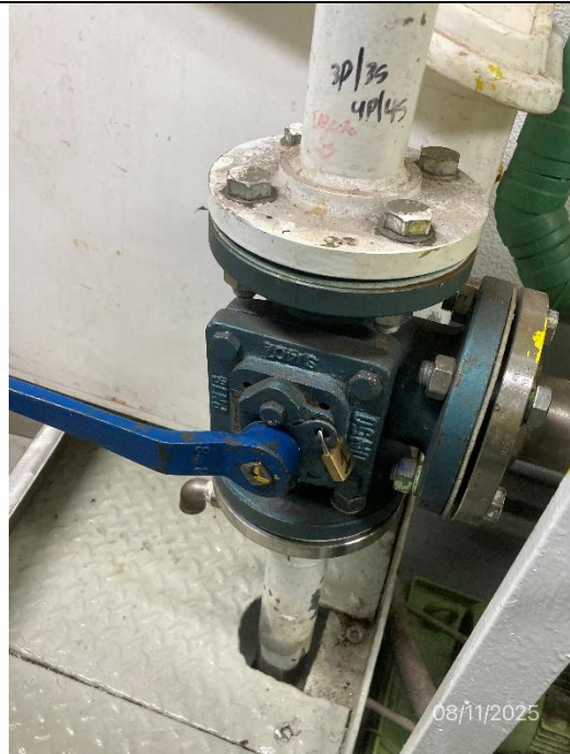
Photo # 6 Image: IMG_2945 Date: 8/11/2025 Taken by: Evan Dobrowski Description: Photo of blackwater MBR discharge valve with padlock.
