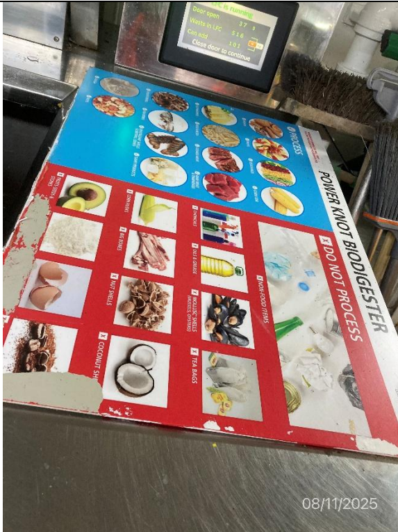
Photo # 17 Image: IMG_2969 Date: 8/11/2025 Taken by: Evan Dobrowski Description: Photo showing food waste biodigester.
