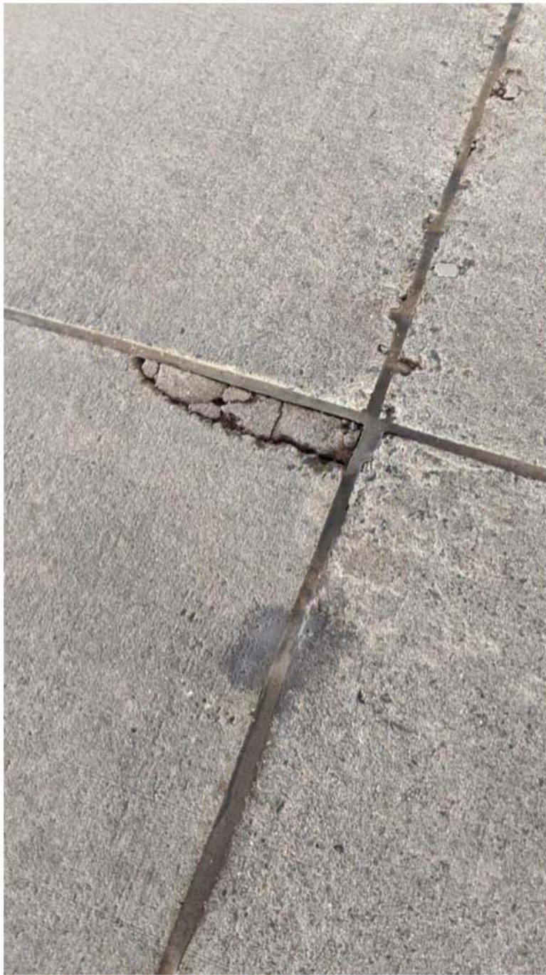
Figure 13 - Deck Crack at Intermediate Joint
