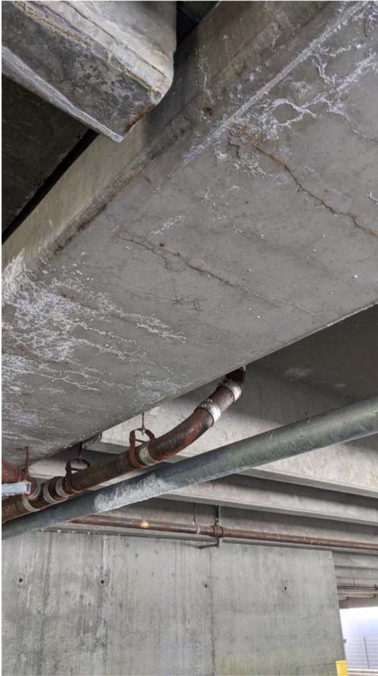
Figure 27 - Severe Cracking with Efflorescence and Rust Staining - Upper Level Girder
