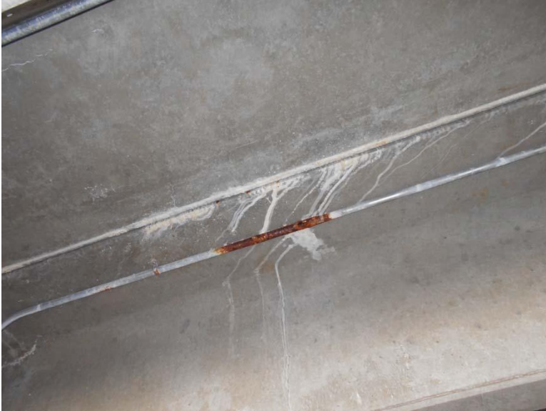
Photograph 29: Efflorescence and corrosion of steel conduit resulting from inward migration of water through concrete structure elements.
