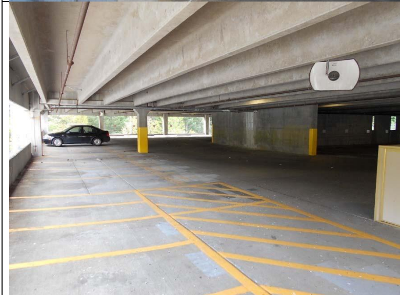
Photograph 5: Overview of the precast double T configuration.
