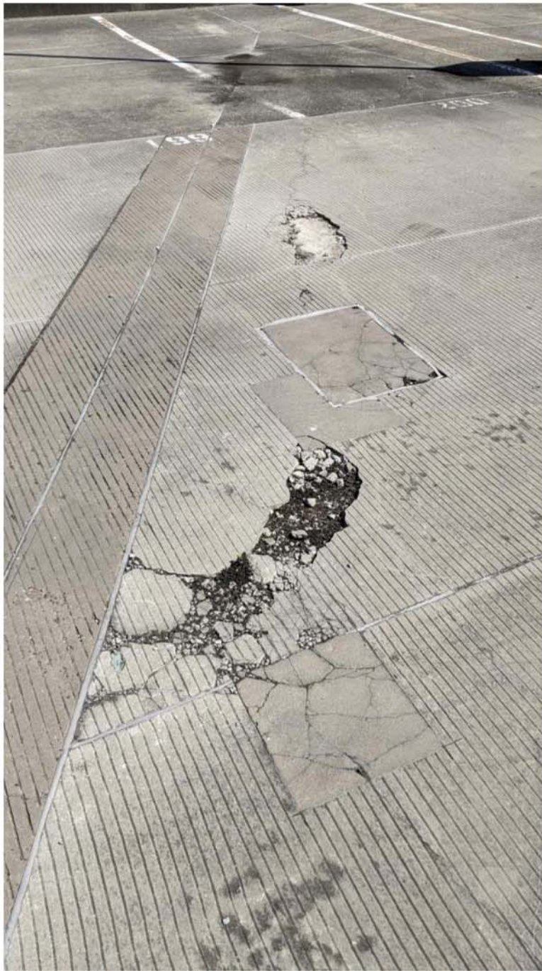
Figure 28 - Cracking, Spalling and Potholes in Upper Level Deck
