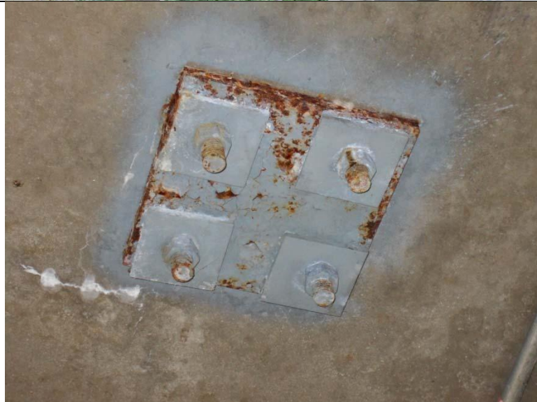
Photograph 9: Detail view from previous image, showing corrosion of the plate. This condition should be addressed at the time of repairs.
