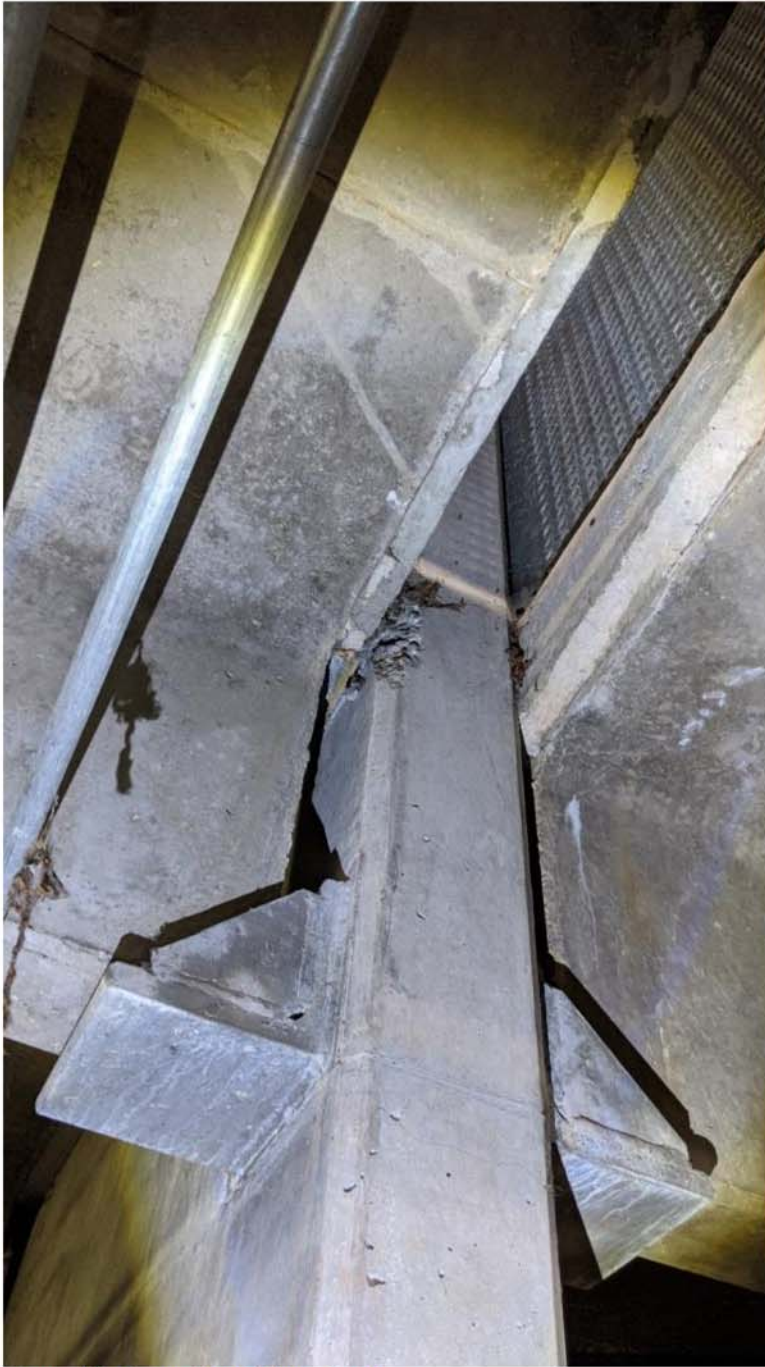
Figure 10 - Center Wall Minor Spalling
