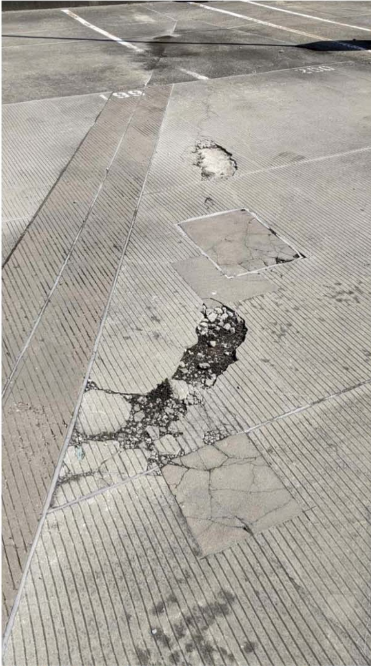
Figure 29 - Cracking, Spalling and Potholes in Upper Level Deck
