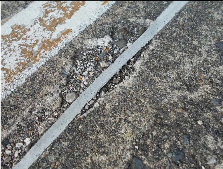
Photograph 16: Detail from previous image showing deterioration of joint edge.
