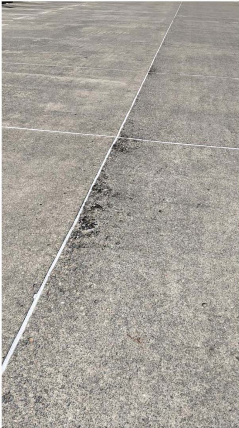
Figure 20 - Deck Spalling and Aggregate Exposure
