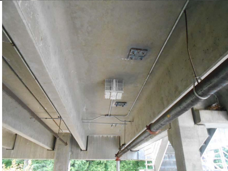
Photograph 8: Steel plates installed at the underside of the deck, south end of level 3.
