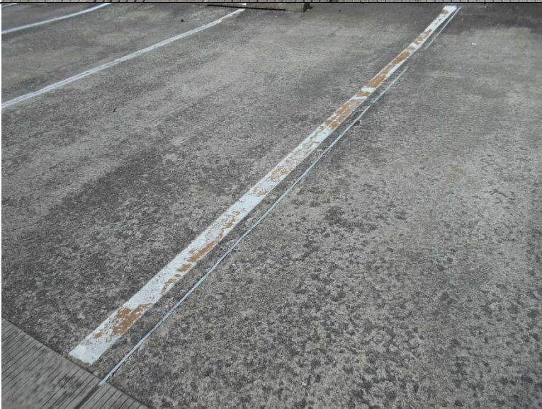
Photograph 15: Typical sealant joint overview.
