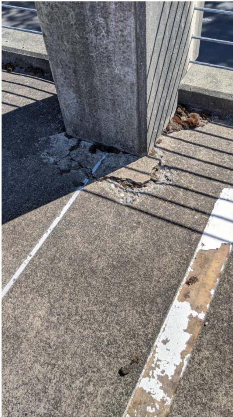
Figure 14 - Deck Cracking at Columns
