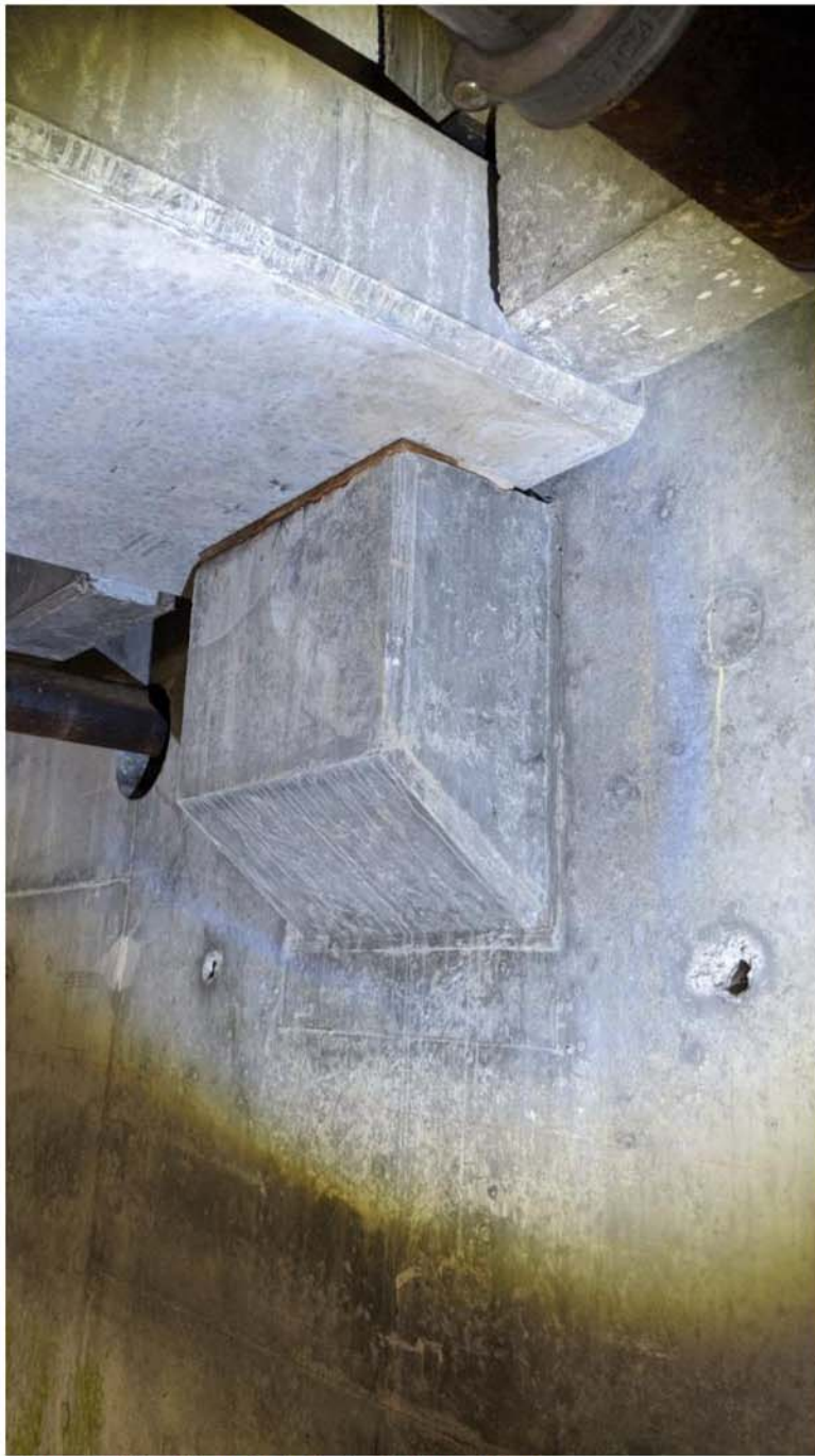
Figure 5 - First Floor Corbel - South End of Garage
