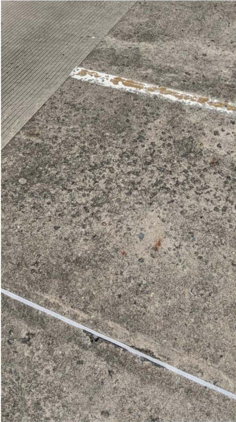
Figure 21 - Deck Aggregate Exposure
