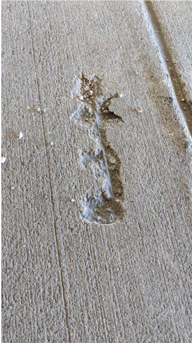
Figure 18 - Minor Deck Spall with Exposed Reinforcing
