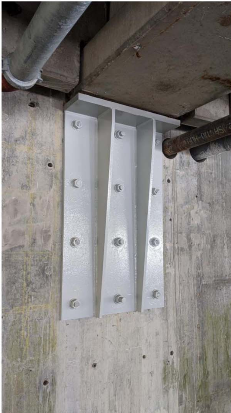
Figure 25 - New North Corbel Supporting Upper Level Girder
