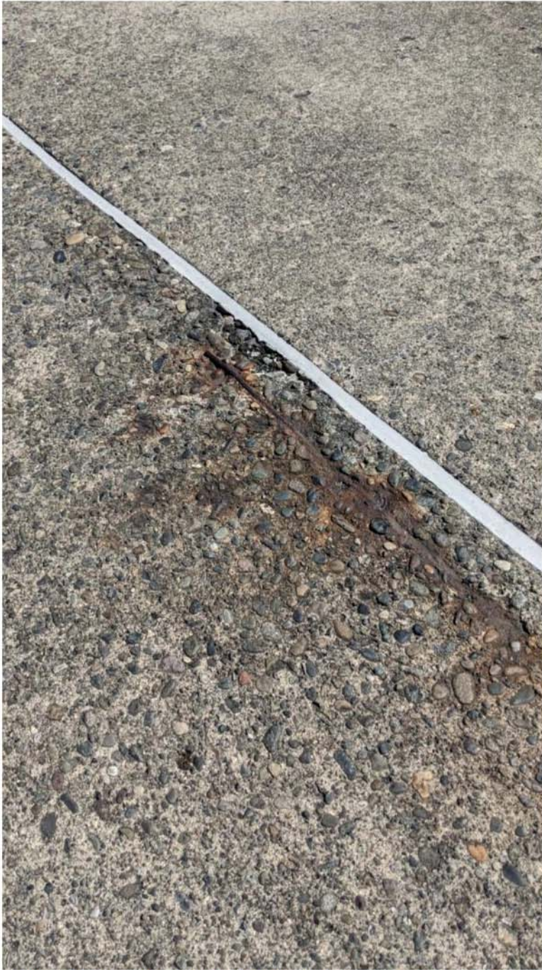
Figure 19 - Exposed, Rusty Reinforcing and Deck Aggregate Exposure
