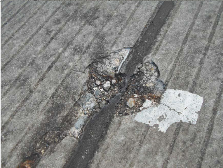
Photograph 18: Detail from previous image showing deterioration of joint edge.
