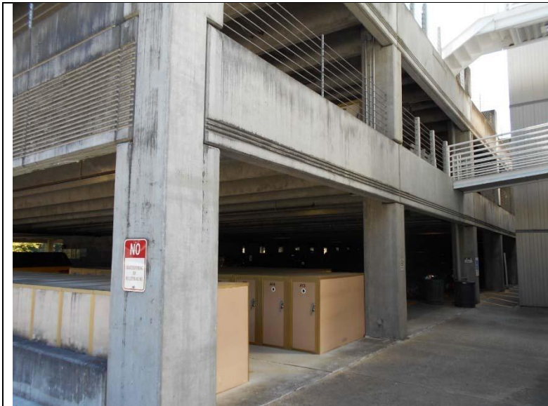
Photograph 4: West elevation overview, showing precast columns and beams.
