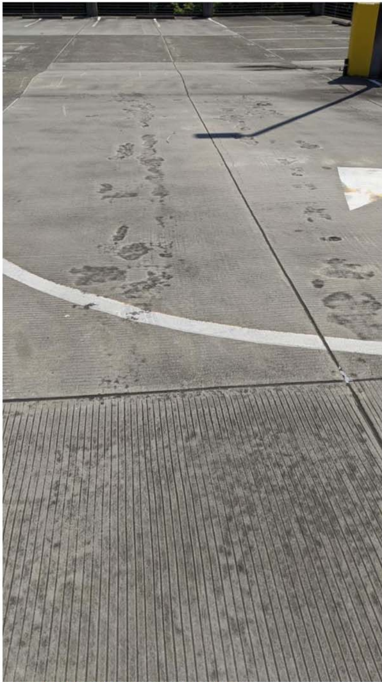
Figure 23 - Water Stained Low Spots in Overlay
