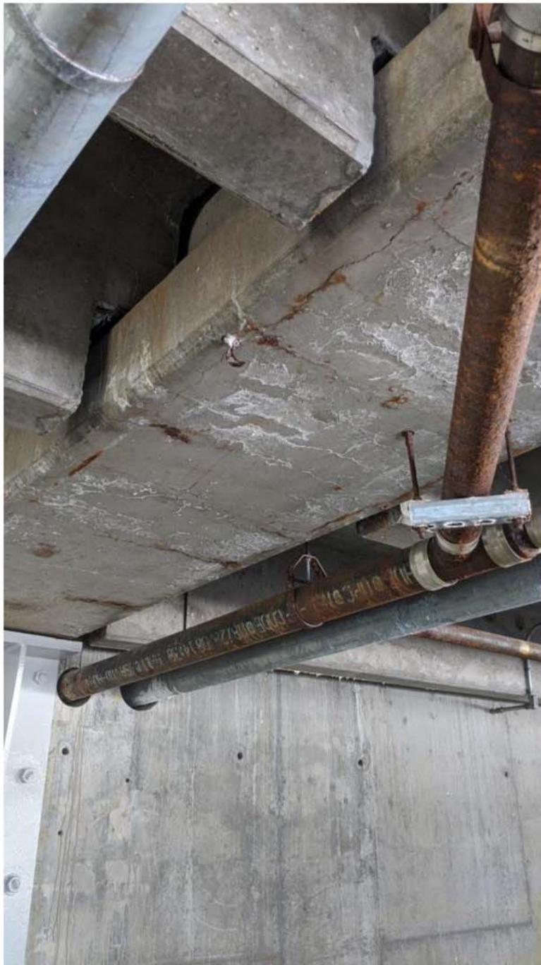
Figure 26 - Severe Cracking with Efflorescence and Rust Staining - Upper Level Girder
