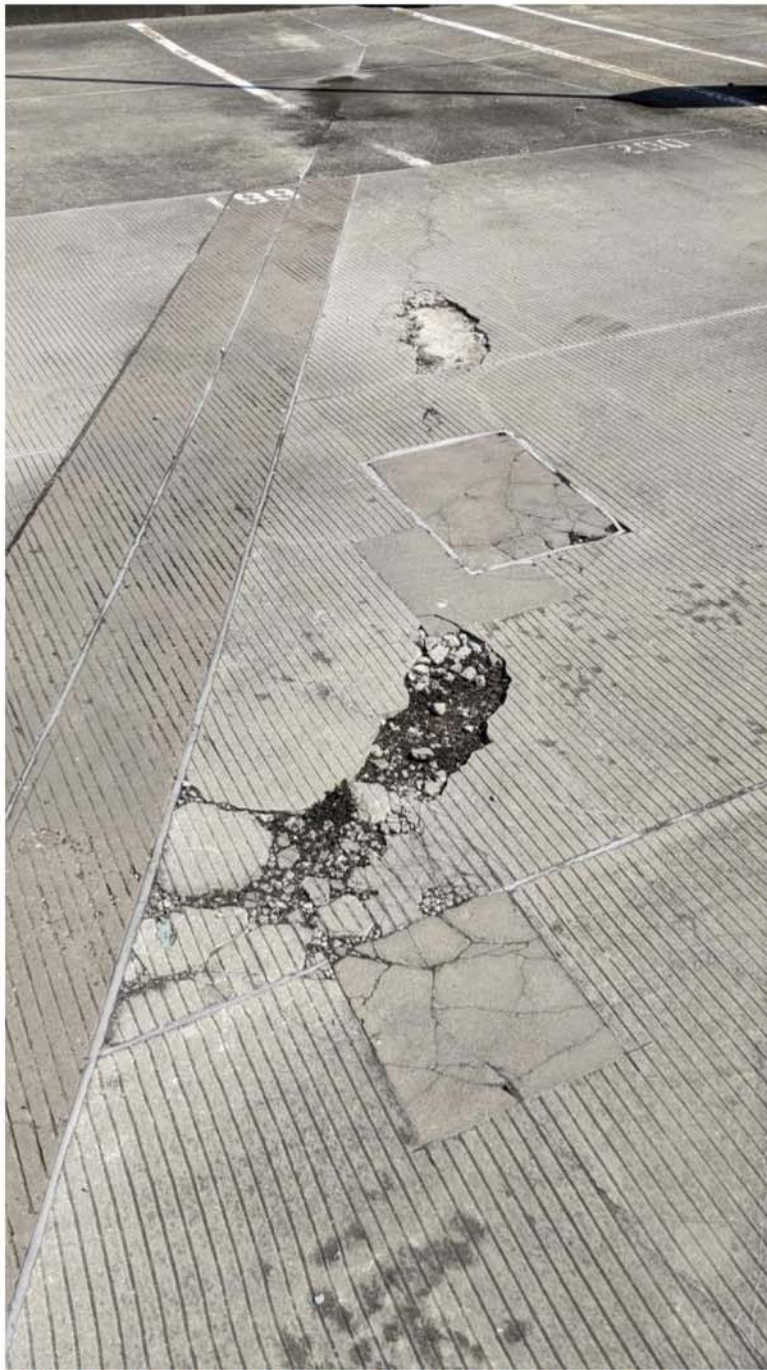
Figure 24 - Cracking, Spalling and Potholes in Upper Level Deck
