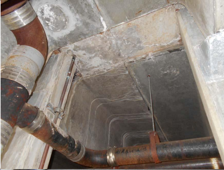
Photograph 28: Efflorescence and corrosion of steel elements resulting from inward migration of water through concrete structure elements.
