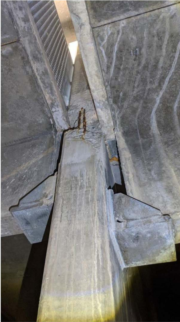
Figure 9 - Center Wall Spall (appears to have been patched and re-spalled)
