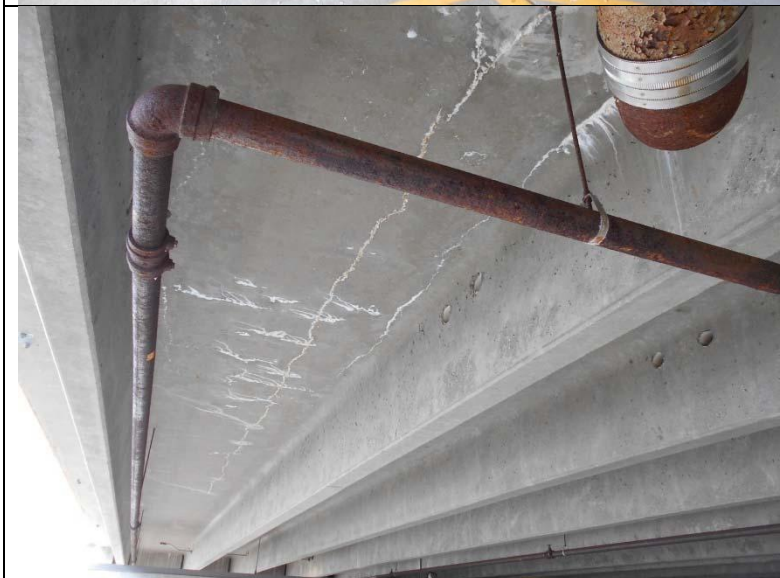
Photograph 6: Detail from previous image showing efflorescence from water migration on the underside of a double T.
