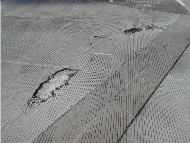
Photograph 14: Detail from photo 12 showing deterioration of the topping layer.
