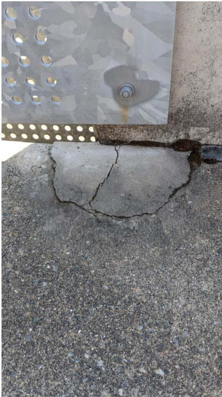
Figure 15 - Deck Cracking at Walls
