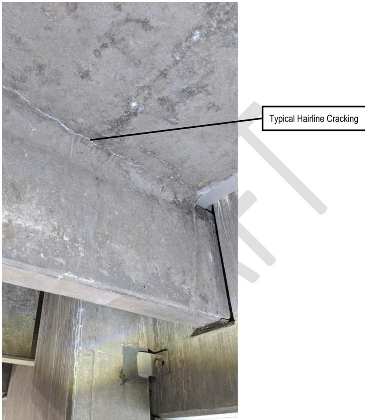
Figure 6 - Typical Hairline Cracking in Double-Tee Beams
