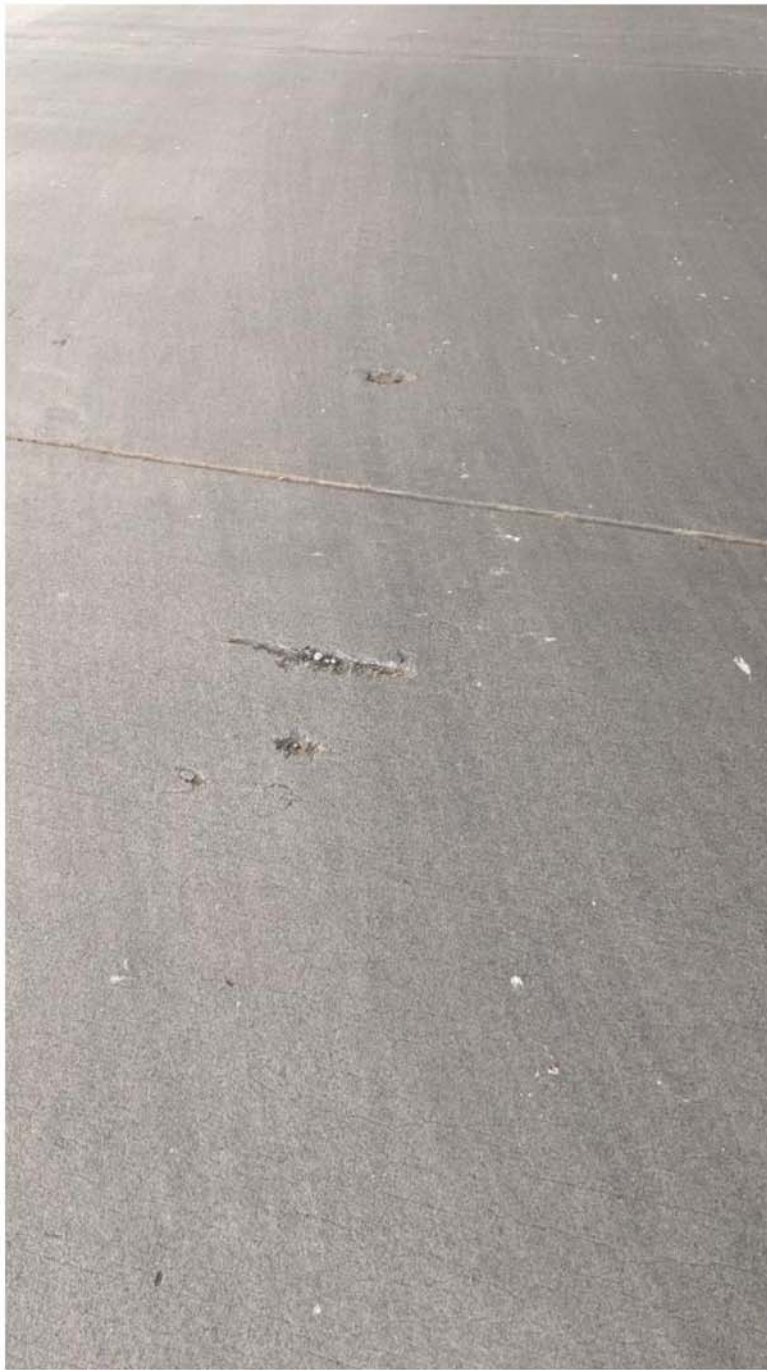
Figure 17 - Minor Spalls in Deck
