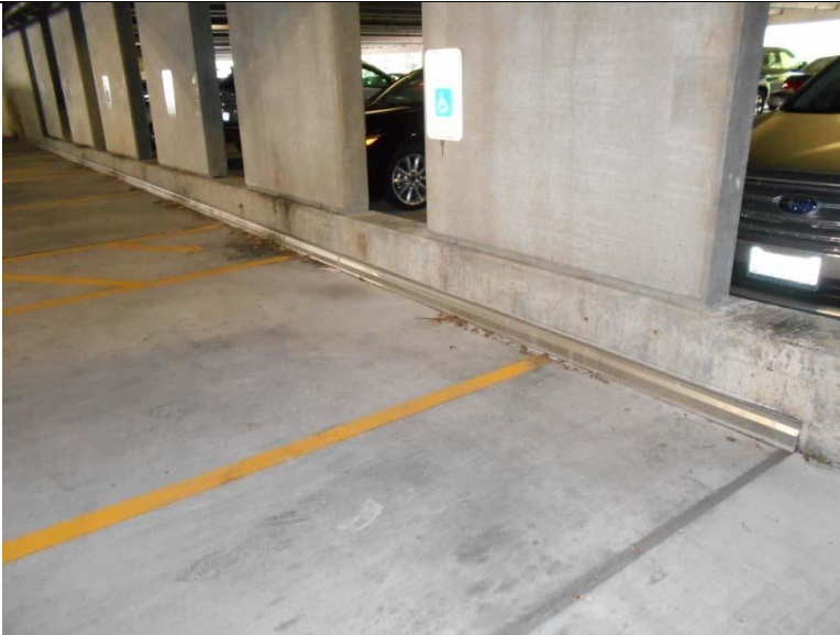
Photograph 10: Sheet metal flashing installed at the interior termination of the topping slab, level 1.
