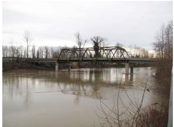
Avenue D bridge over Snohomish River
