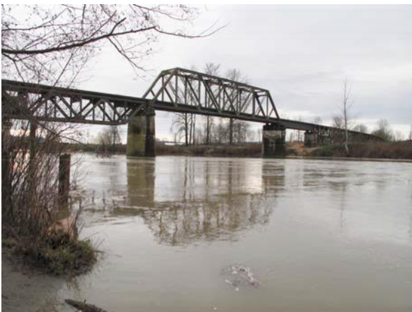
Railroad trestle bridge
