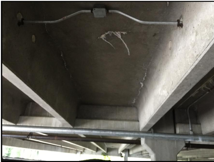
**Photo 3:** Cracks forming in the structural members of the top parking deck. Continued water intrusion causes the cracks to grow weakening the structure and will eventually cause failure of the structure.
