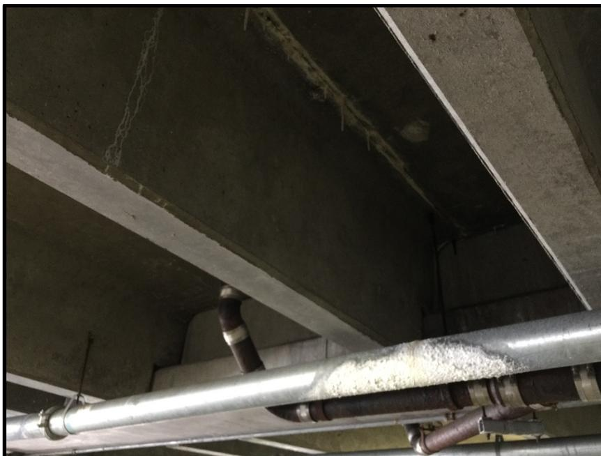
**Photo 2:** The bright colored pipe is part of the fire sprinkler system and was replaced recently due to corrosion from the leaks. Also cracks in the structural elements of the garage are forming and growing due to the water intrusion.
