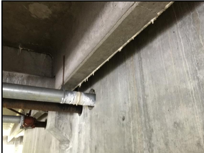
**Photo 1:** Water seeping through the concrete upper parking deck washing the minerals out of the structural concrete elements weakening the overall structure.
