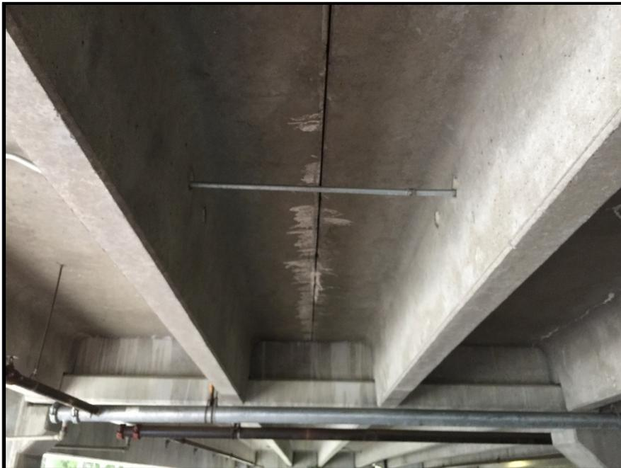
**Photo 4:** Joints between precast structural members showing water intrusion. Continued intrusion. Will cause failure of the joint.
