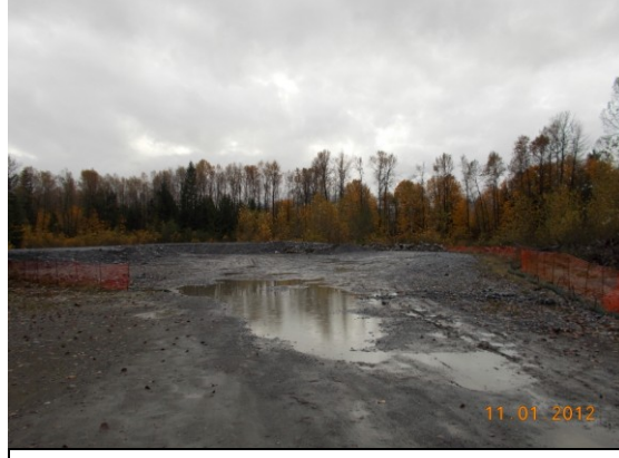
Photo 6 (Segment 3) View west showing access to permitted temporary rock storage area adjacent to right bank of Baker River.
