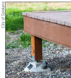
MINIMAL EXCAVATION FOUNDATIONS
