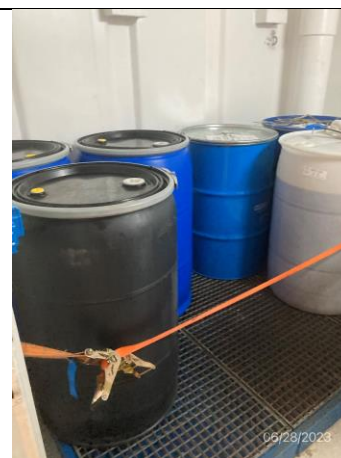
Photo #09 6/28/23 Image: IMG_E394 By: Dobrowski Description: barrel storage with used cooking oil and various other waste chemicals.
