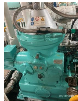
Photo #05 6/268/23 Image: IMG_E414 By: Dobrowski Description: OWS oil treatment
