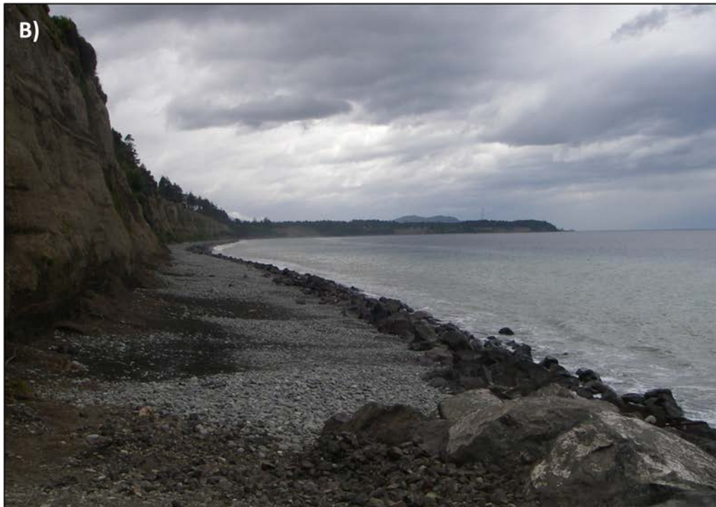
Figure 3. A) Photograph of the Dungeness bluffs looking west from Dungeness Spit. B) Photograph of the Elwha bluffs west from Ediz Hook. Note the armoring placed mid-beach in front of the bluffs.
