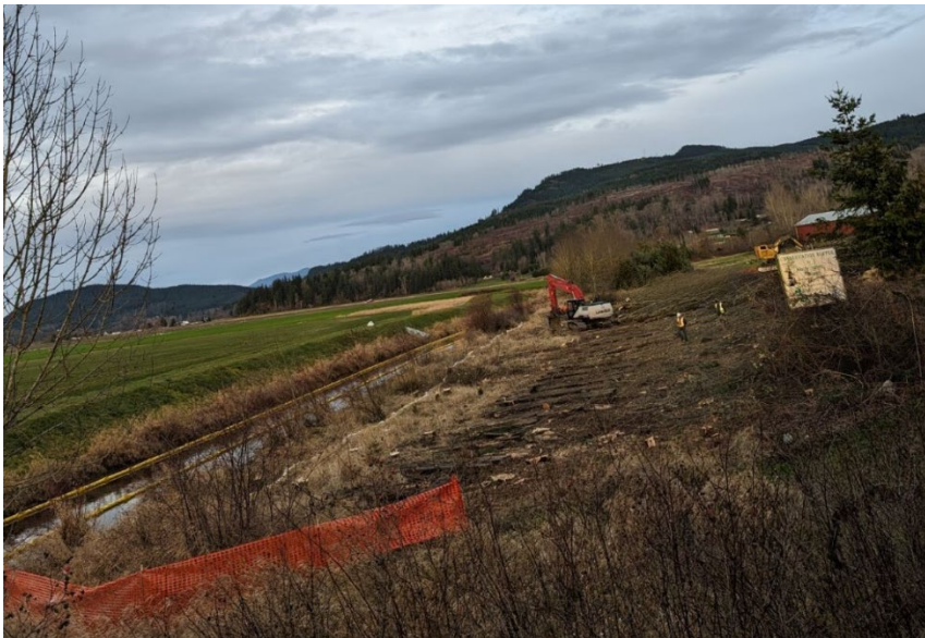
Tree removal area adjacent to Hill Ditch.
