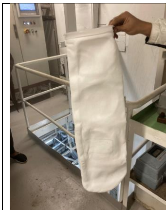
Photo #11 5/8/23 Image: IMG_213 By: Dobrowski Description: Wet Scrubber filter
