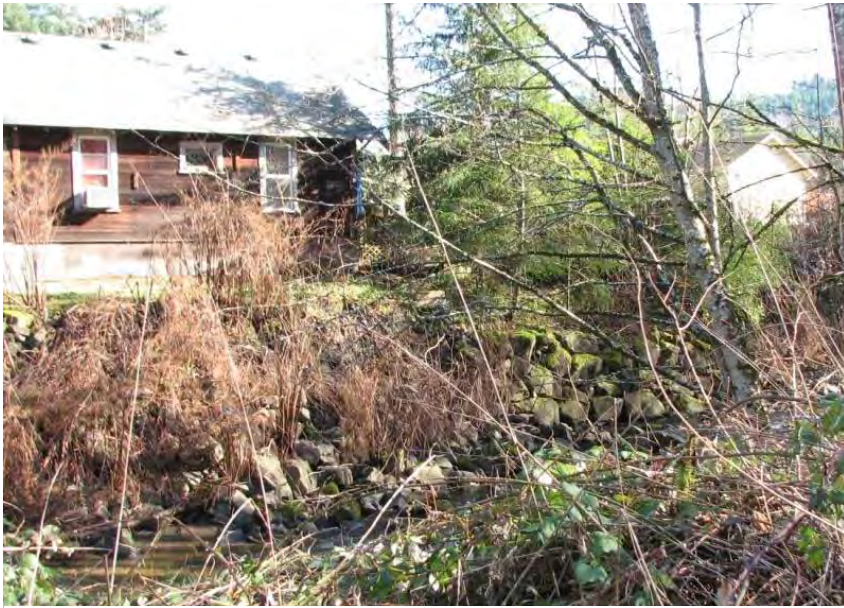
Photo 5: Reach 1c: Photo on left is incised channel in Reach 1c. Riprap is evident on stream right. Some is failing.
