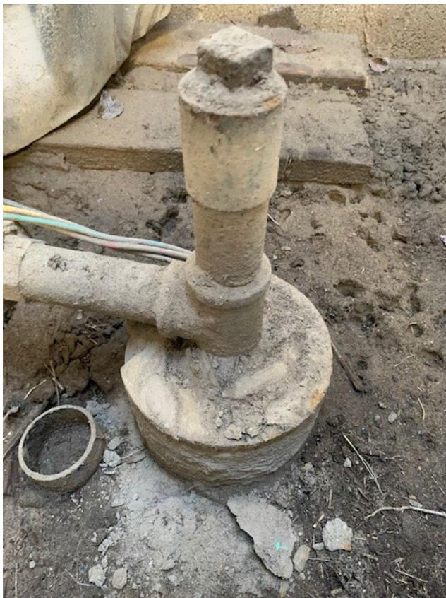
**Figure 11. Wellhead for ZIL-04.**
