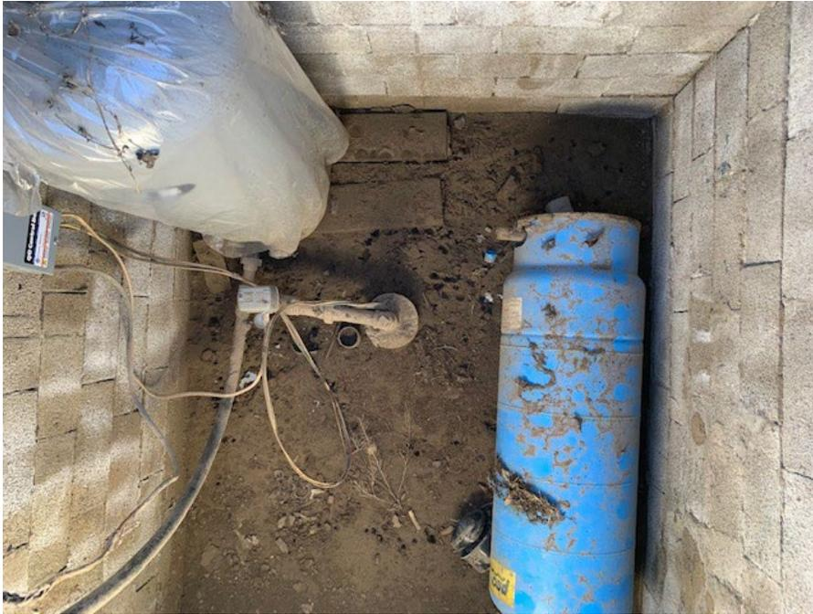
**Figure 10. View of pit, pressure tank, and wellhead for ZIL-04.**
