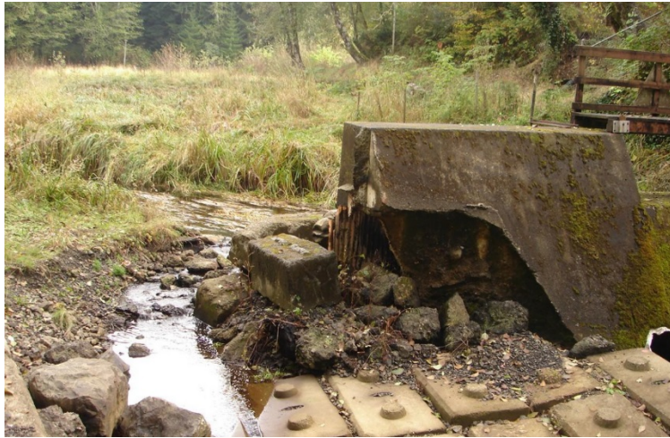
Mill Creek Dam Breach in Mill Creek Reach.
