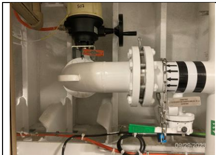
Photo #11 9/29/23 Image: IMG_E0732 By: Dobrowski Description: overboard discharge lock
