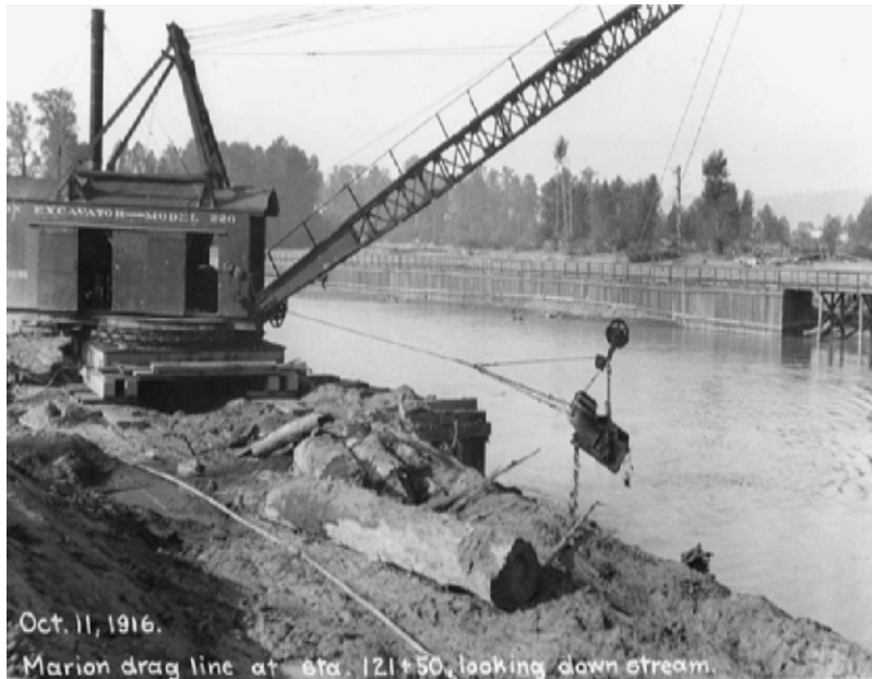
Photograph 3-2. Marion drag line and dredging along the Puyallup River during channel straightening dated October 11, 1916 (Pierce County River Improvement District, 1991).
