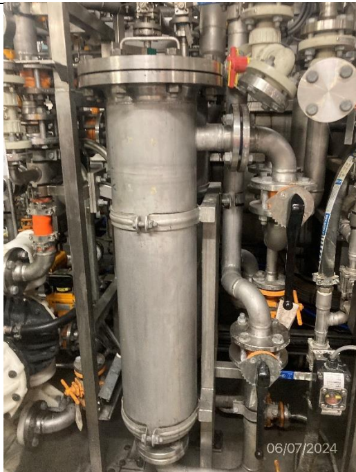
Photo # 43 Image: IMG_1714 Date: 6/7/2024 Taken by: Evan Dobrowski Description: EGCS filter housing
