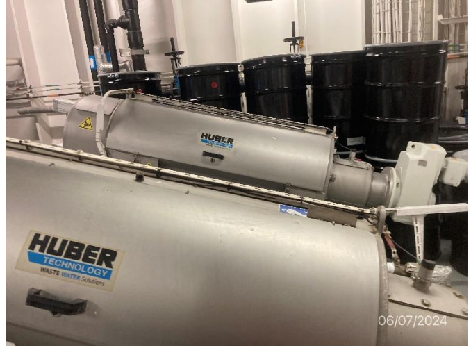
Photo # 50 Image: IMG_1721 Date: 6/7/2024 Taken by: Evan Dobrowski Description: Bio Sludge Dewatering press
