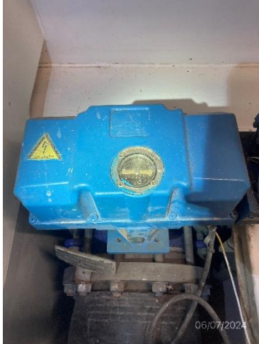
Photo # 33 Image: IMG_1704 Date: 6/7/2024 Taken by: Evan Dobrowski Description: Sewage overboard valve in the closed position
