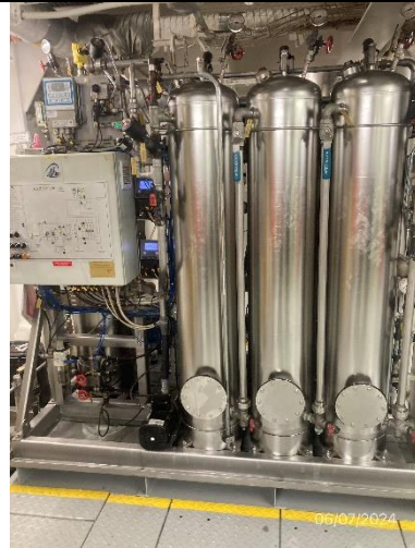
Photo # 26 Image: IMG_1697 Date: 6/7/2024 Taken by: Evan Dobrowski Description: Bilge water filters.
