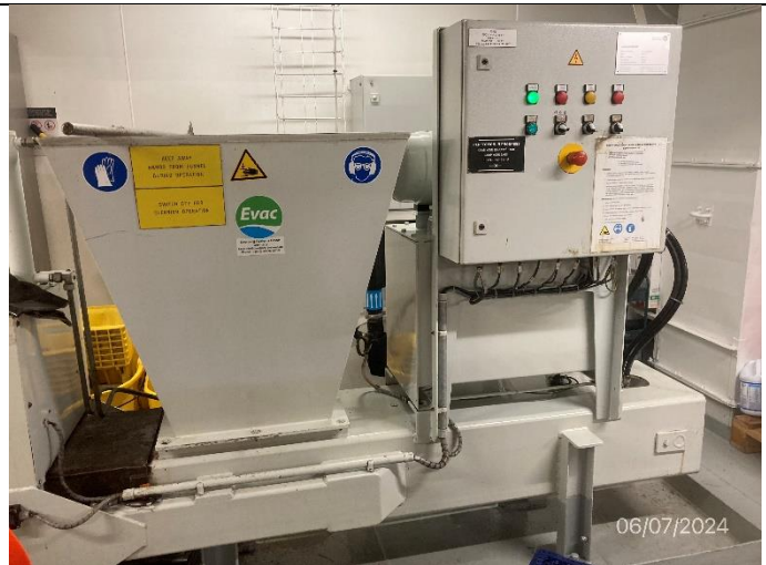
Photo # 50 Image: IMG_1721 Date: 6/7/2024 Taken by: Evan Dobrowski Description: Bio Sludge Dewatering press
