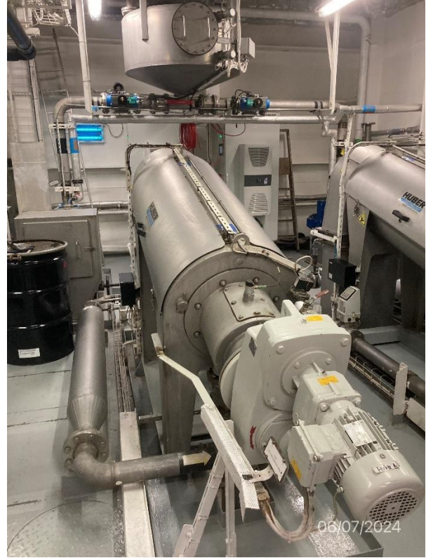
Photo # 46 Image: IMG_1717 Date: 6/7/2024 Taken by: Evan Dobrowski Description: Bio Sludge Dewatering press
