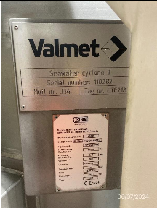
Photo # 41 Image: IMG_1712 Date: 6/7/2024 Taken by: Evan Dobrowski Description: Valmet Seawater Cyclone – Part of EGCS system.
