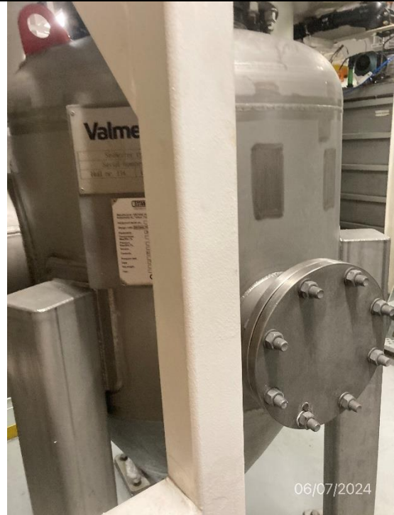
Photo # 42 Image: IMG_1713 Date: 6/7/2024 Taken by: Evan Dobrowski Description: Valmet Seawater Cyclone – Part of EGCS system.
