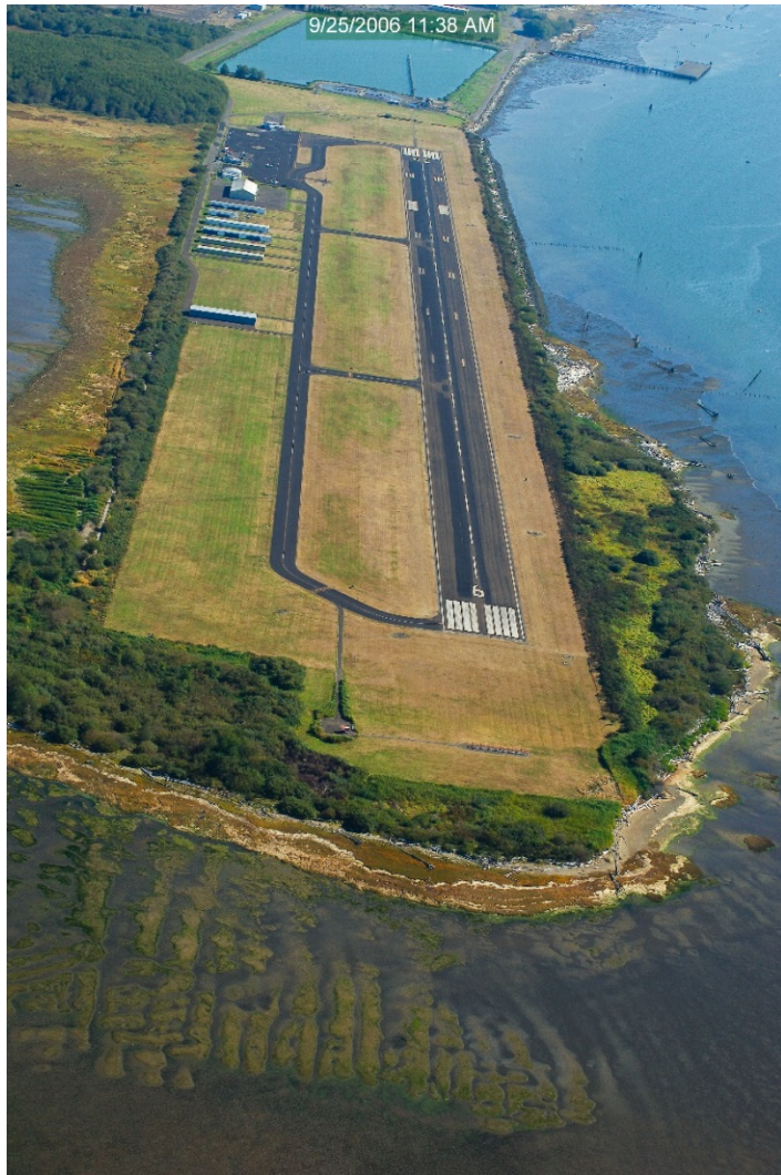
Fill at Bowerman Airport in Grays Harbor Reach in Hoquiam.
