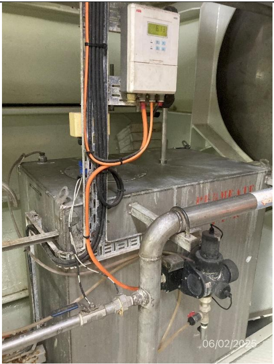
Photo # 5 Image: IMG_2805 Date: 6/2/2025 Taken by: Evan Dobrowski Description: Photo of permeate tank
