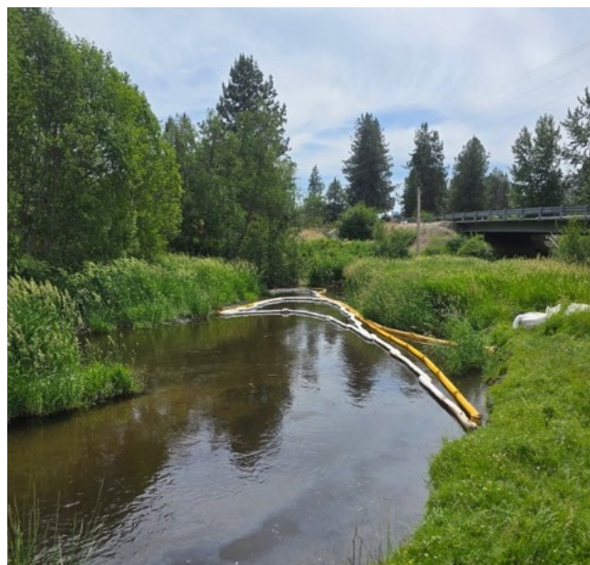
Containment boom is used to isolate the spill along the Little Spokane River.
