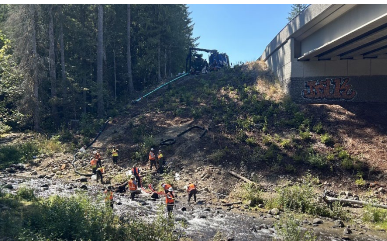
Crews work in Indian Creek near bridge, using a vac truck to remove fuel.
