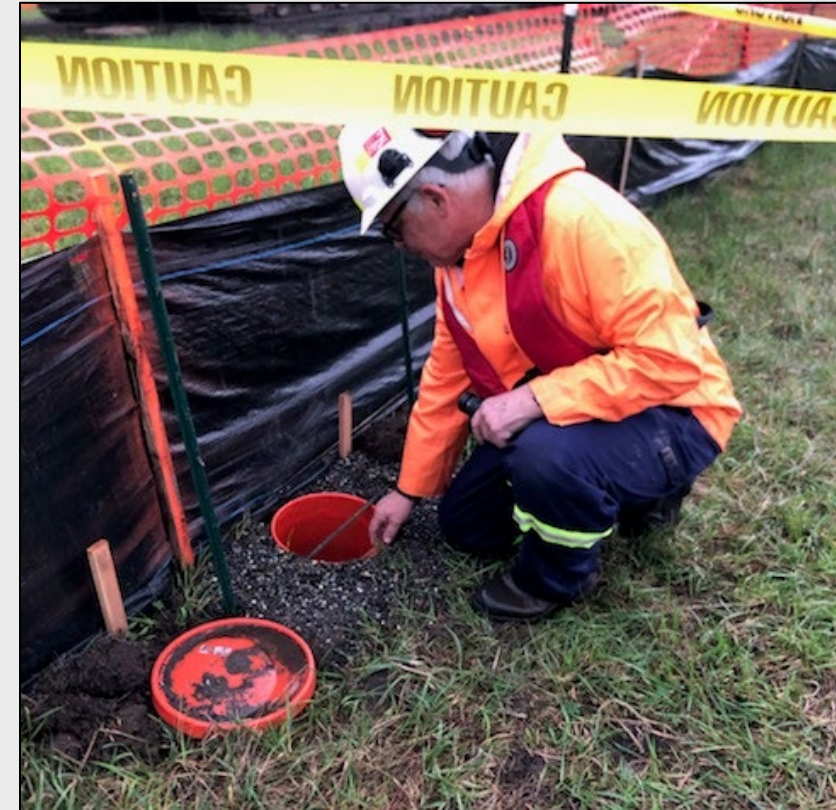
(Wildlife specialist monitors amphibian traps on perimeter of excavation site)
