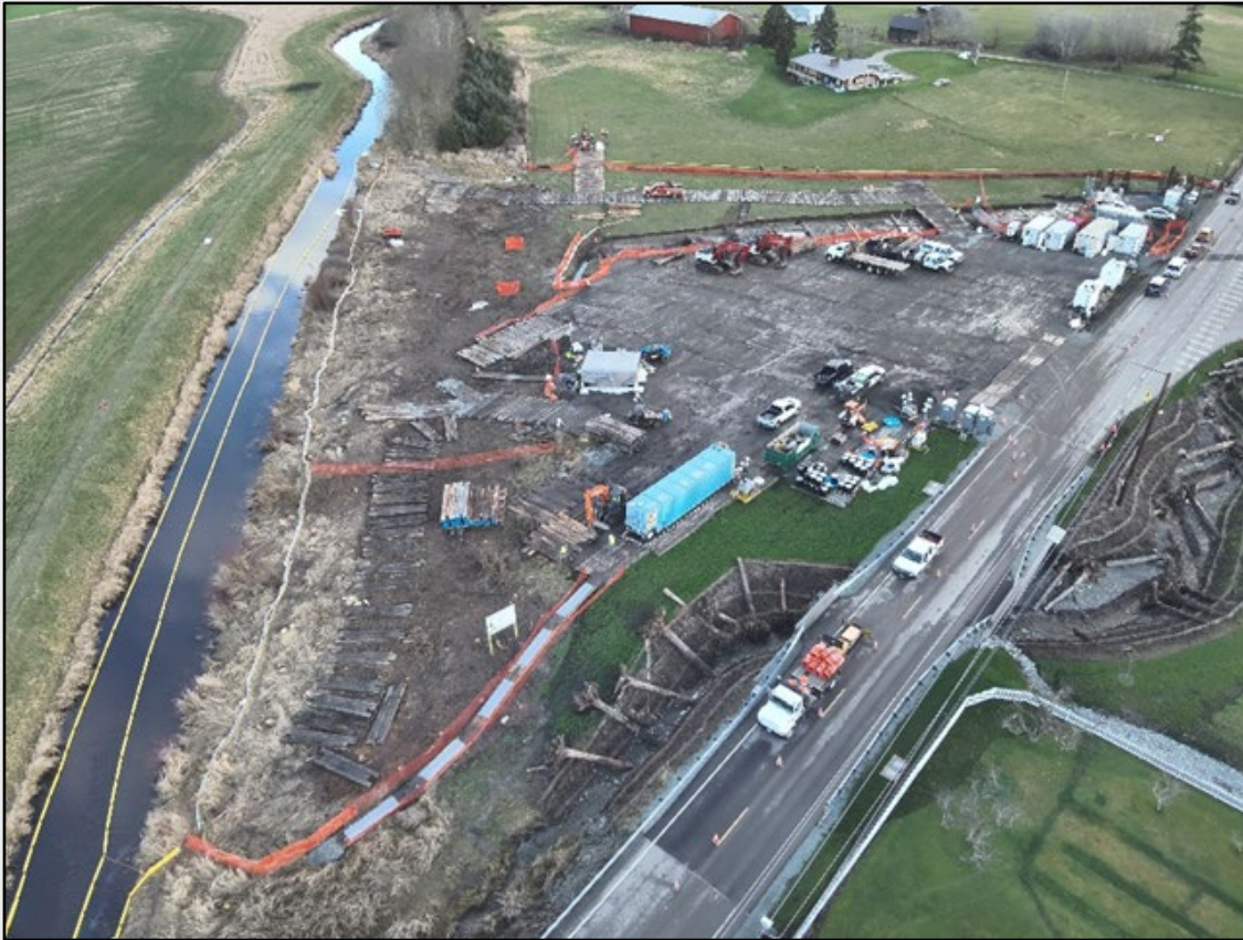
Aerial image of incident site looking West.
