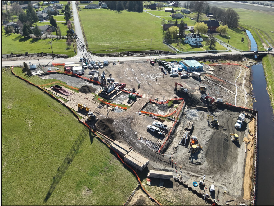
Aerial drone image of incident location facing South.
